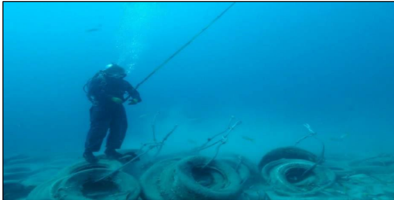
Image 9. Surface air supplied diver hand bundling tires for transport to the surface by crane (Photo: Industrial Divers Corporation [IDC]).
