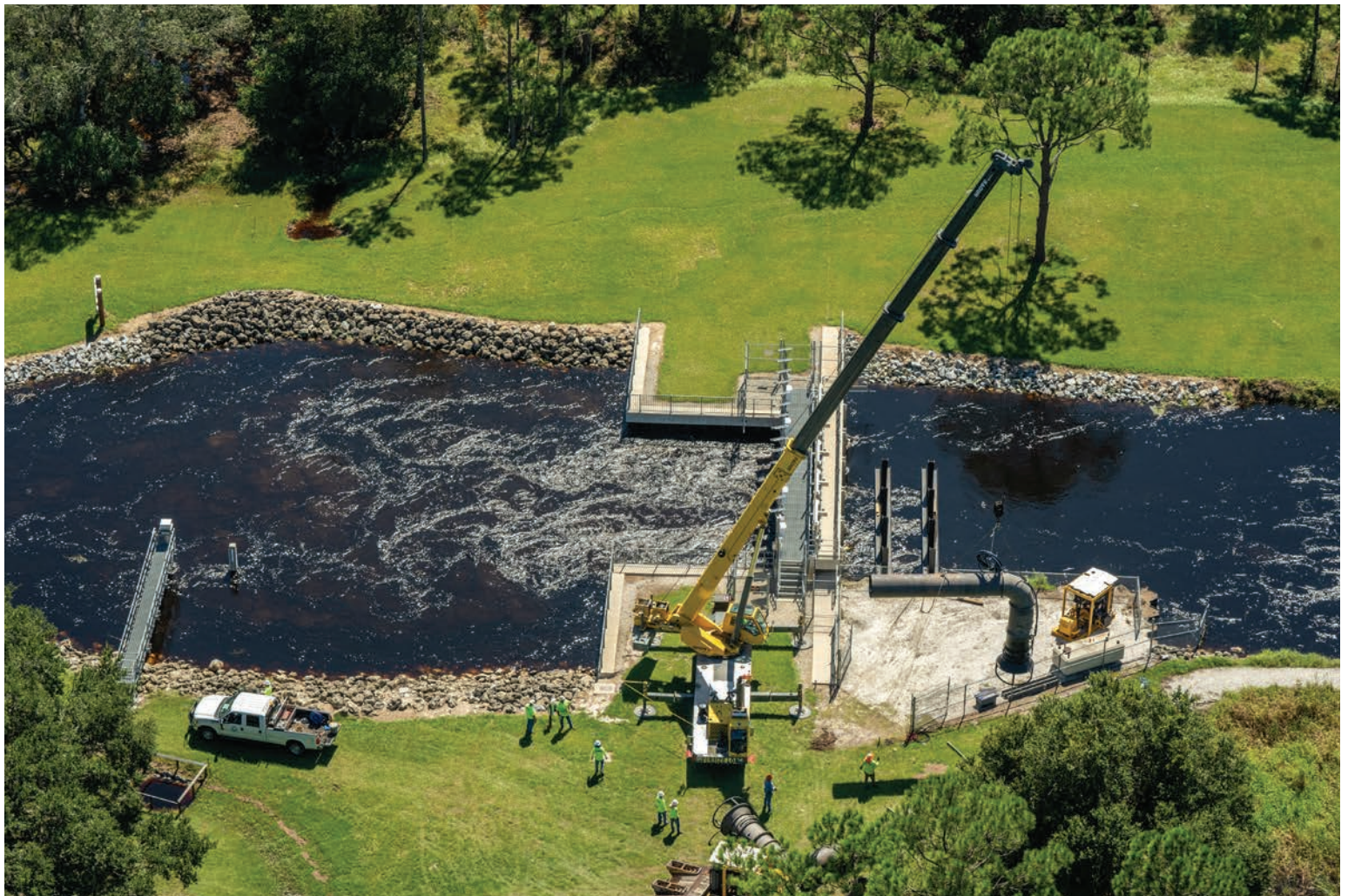
G-103 Structure after Hurricane Ian
