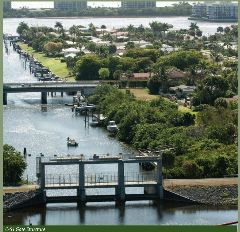
C-51 Gate Structure
