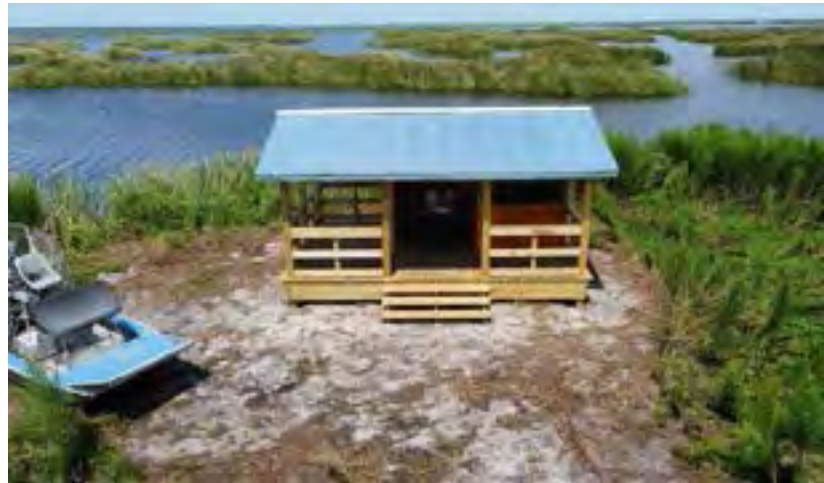
An inclement weather shelter constructed in the Fellsmere Water Management Area.
