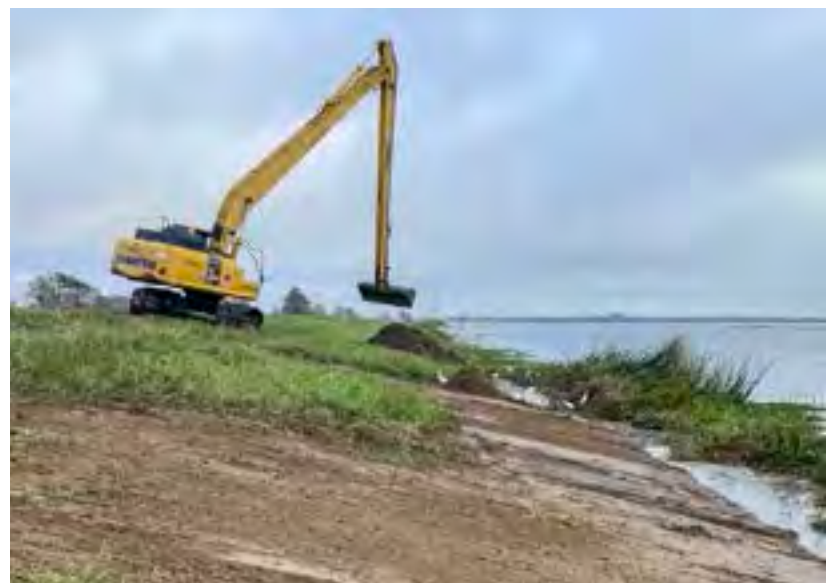
Repair work on the L-77W levee.
