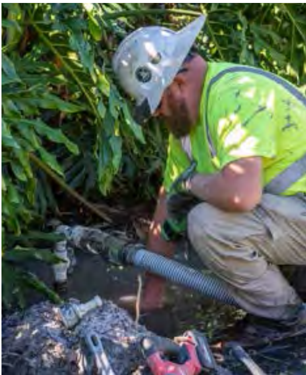
A contractor plugs a free-flowing residential well in Sanford.
