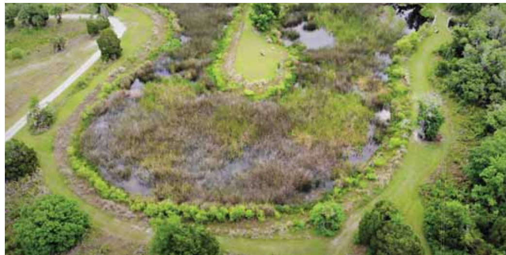
Three Sisters Springs Wetland Treatment Project in Crystal River.
