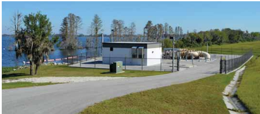
Lake Hancock Outfall Treatment Facility.
