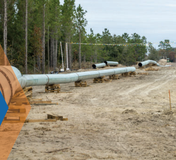
New natural gas pipelines being installed in Gilchrist County.
