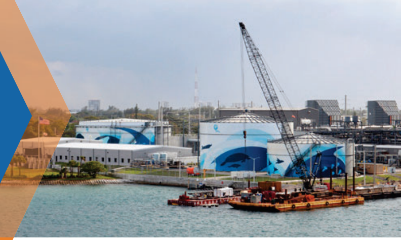
Florida Power & Light storage tanks sit along Manatee Lagoon in West Palm Beach at this natural gas plant. Photo taken May 2018.
