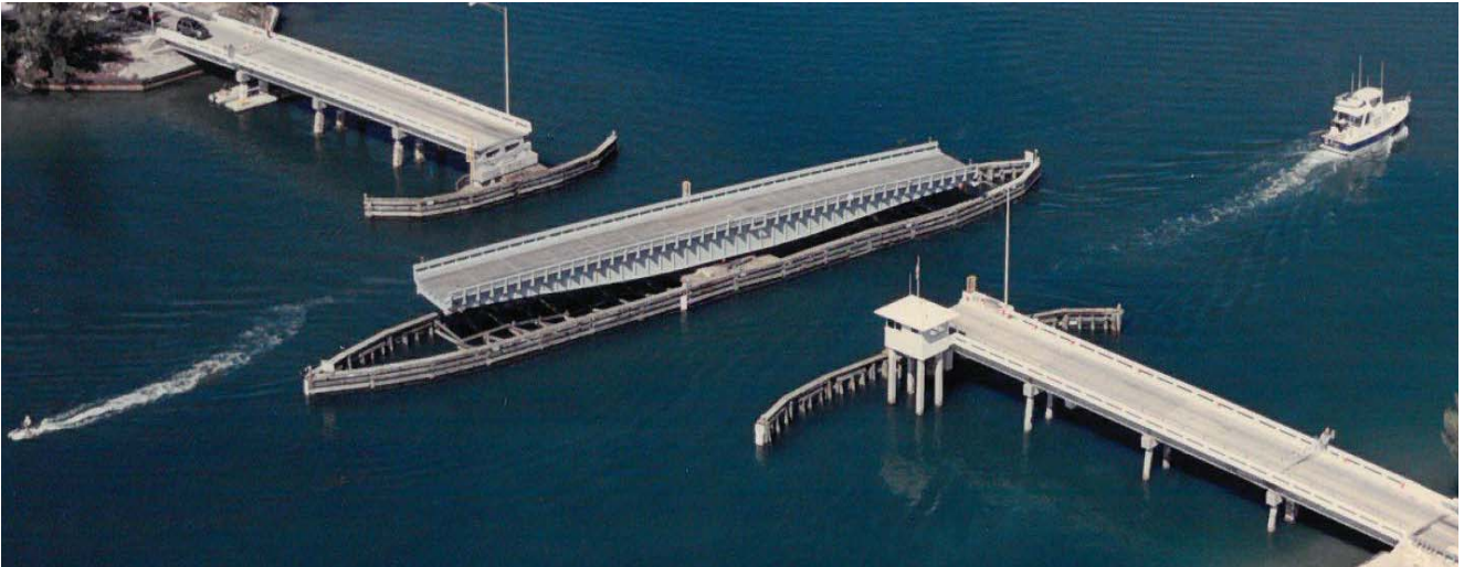
Photo courtesy of Gasparilla Island Bridge Authority
