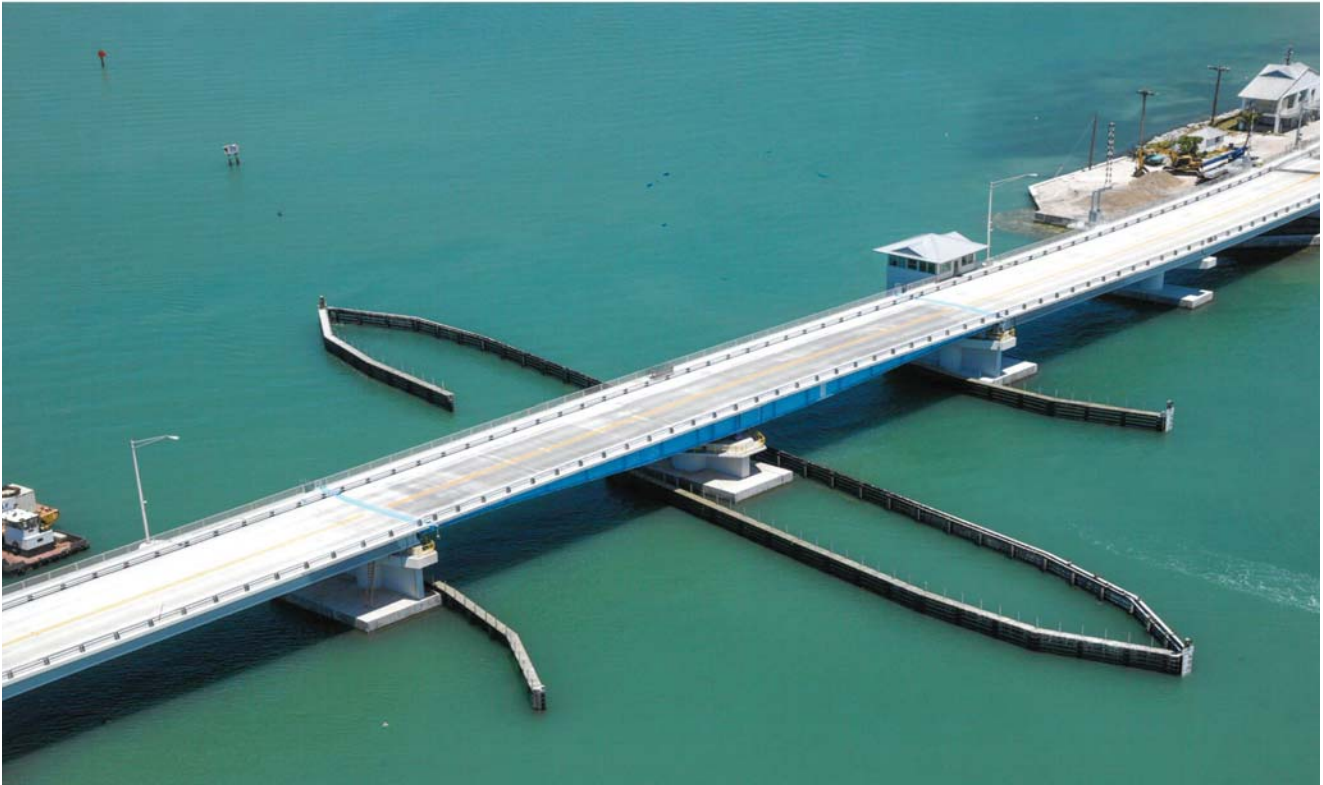
Photo courtesy of Gasparilla Island Bridge Authority
