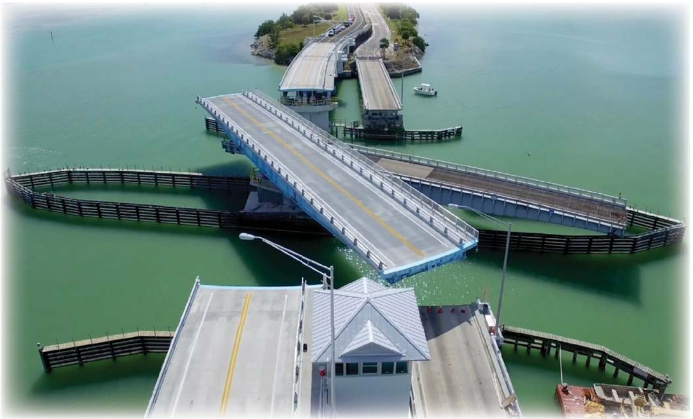
Photo courtesy of Gasparilla Island Bridge Authority
