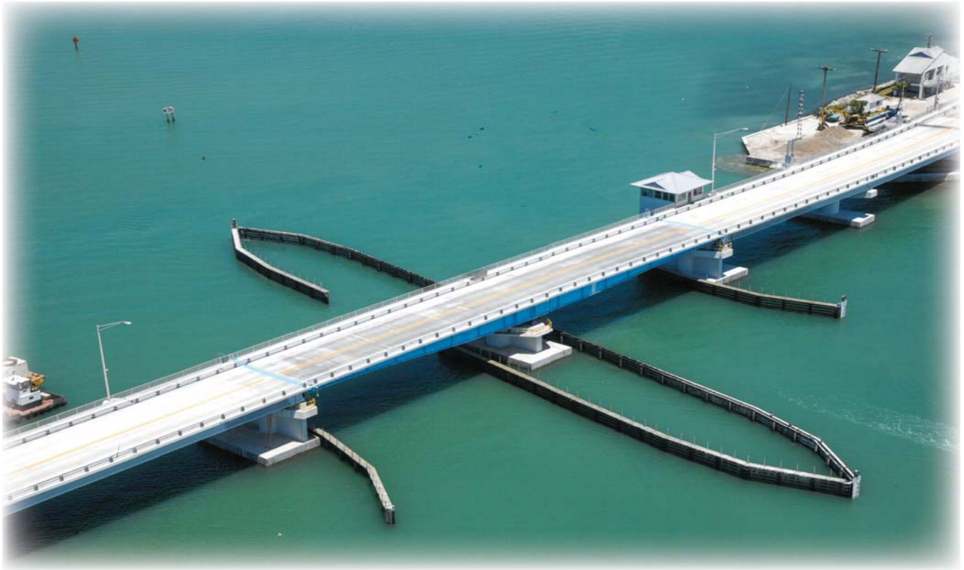
Photo courtesy of Gasparilla Island Bridge Authority
