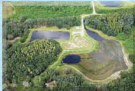
Eastshore Commerce Park Stormwater Hillsborough Co.
