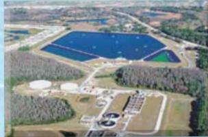
Pasco Wet Weather Reservoir
