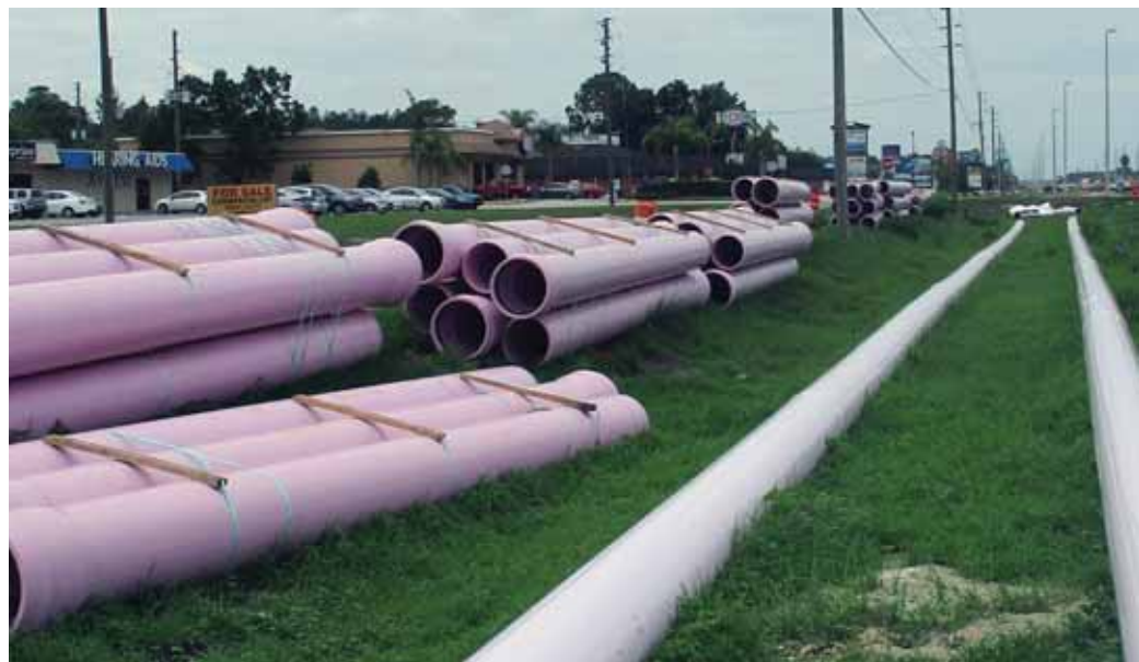
Reclaimed water transmission line construction project on U.S. 19 in Hernando County.
