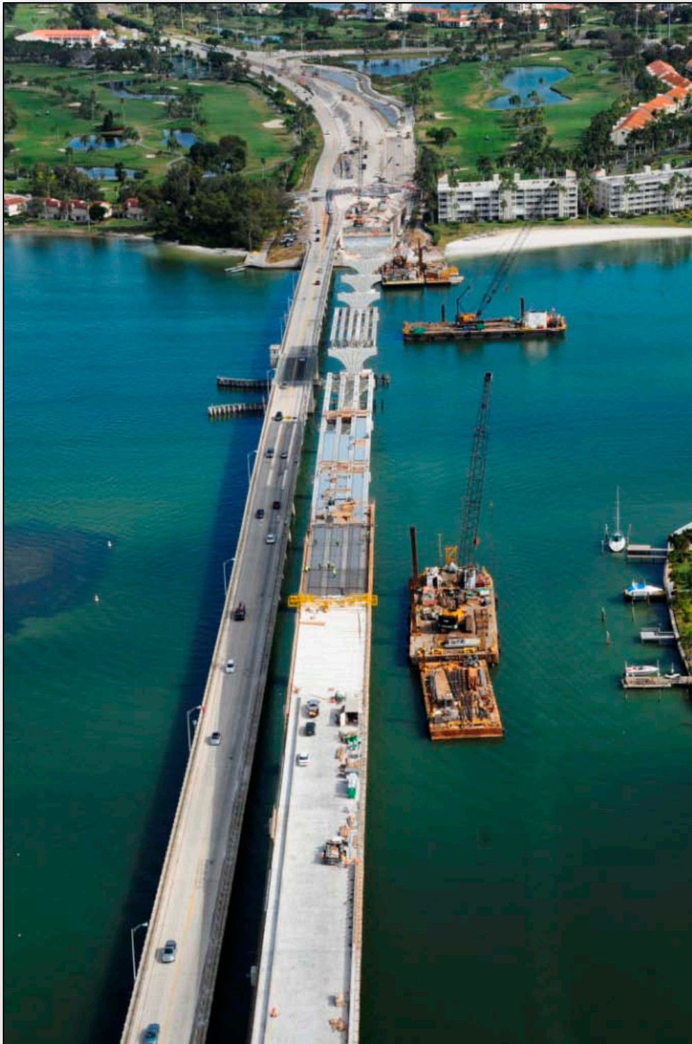
Pinellas Bayway Bridge Replacement in Pinellas County.
