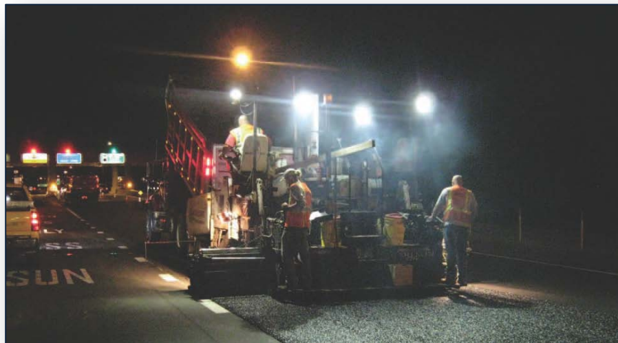
Resurfacing the Southern Connector Extension of Florida's Turnpike.
