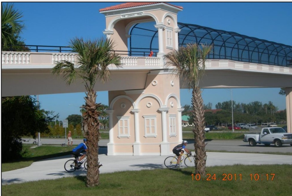
Legacy Trail Pedestrian Bridge in Sarasota County.
