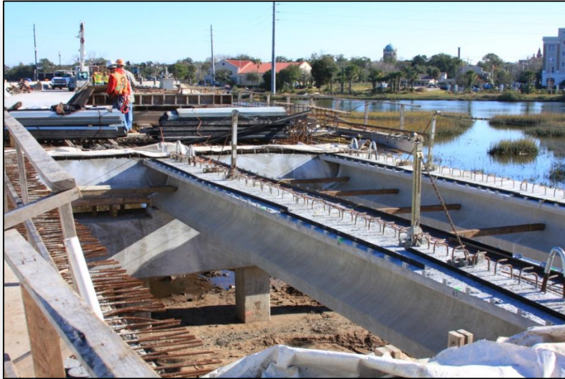
San Sebastian River Bridge Replacement in St. Johns County.
