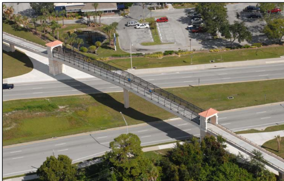
Legacy Trail Pedestrian Bridge in Venice.
