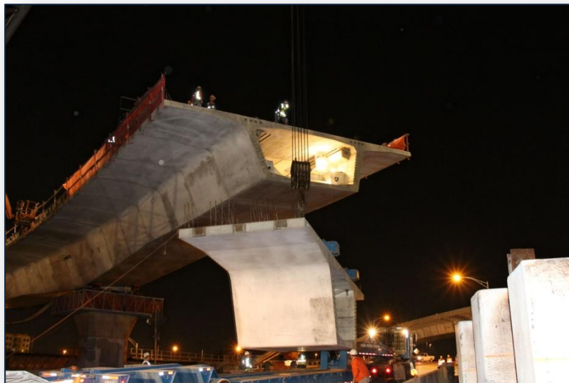
Erection of Bridge Segments for the SR 836/SR 826 Segmental Bridge.
