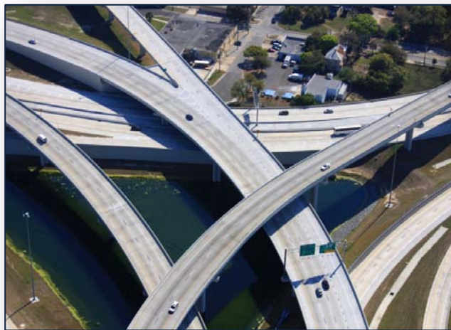
The AASHTO Award Winning Interstate 95/10 Interchange Project in Jacksonville.
