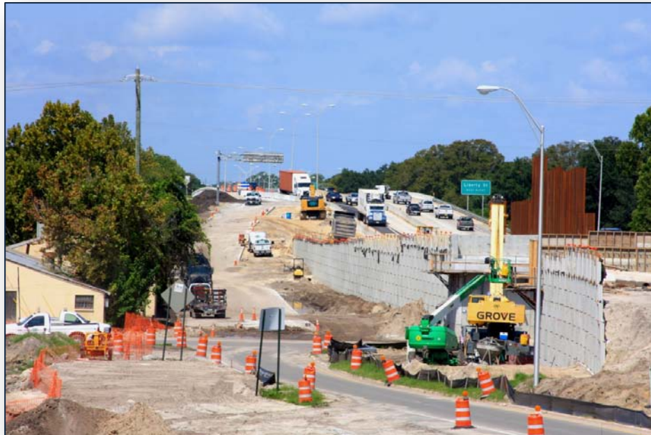
Martin Luther King Parkway/21st Street Interchange Improvements in Jacksonville.
