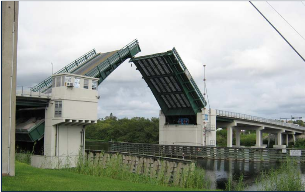
Rehabilitation of the La Belle Drawbridge over Caloosahatchee River.
