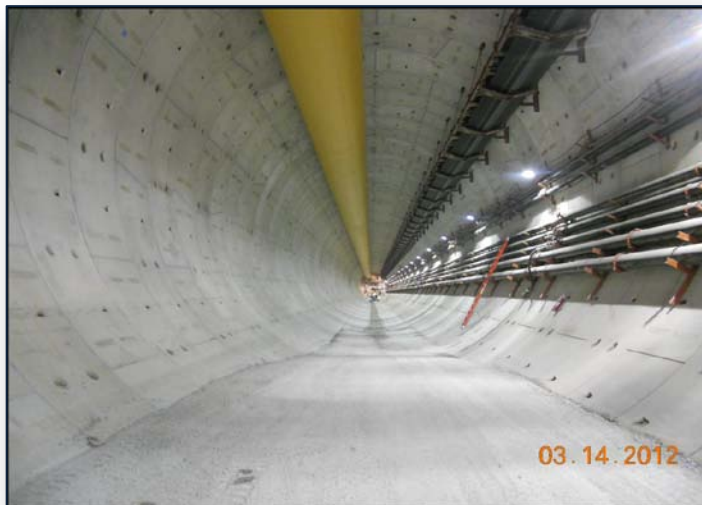
Inside the Port of Miami Tunnel.
