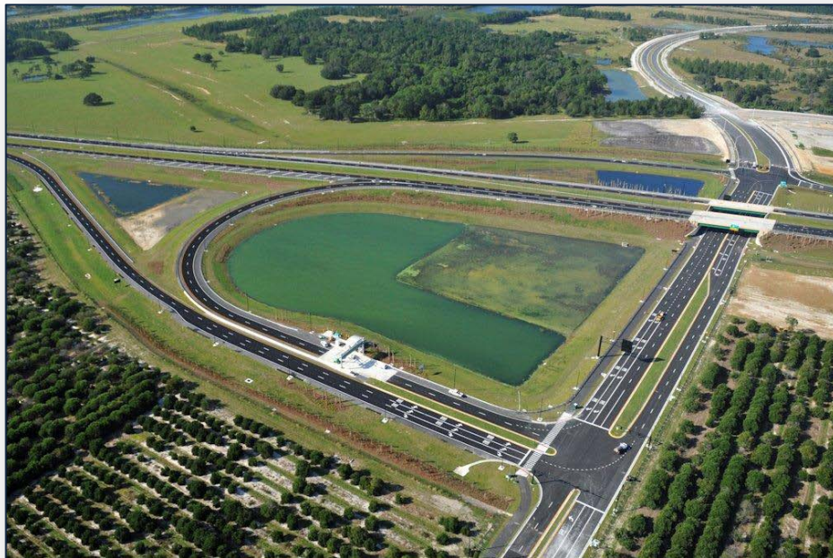
New Pace Road Interchange on the Polk Parkway.
