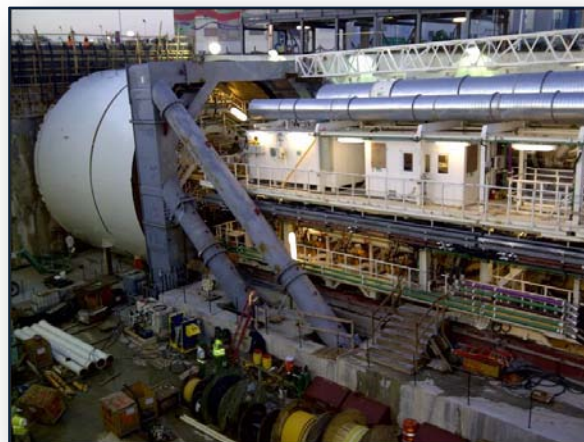
Port of Miami Tunnel Boring Machine Trailing Gear.
