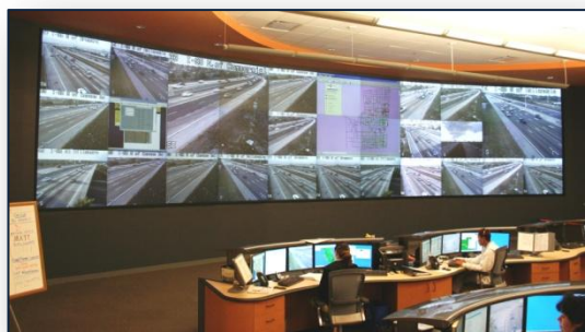
Broward County Traffic Management Center video wall.
