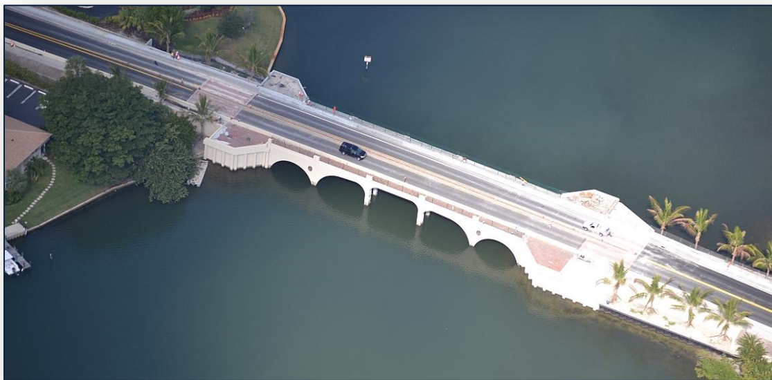
Newly reconstructed Tequesta Bridge in Palm Beach County.
