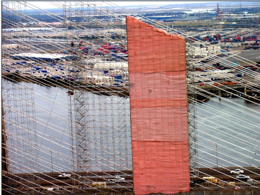
Dames Point Bridge rehabilitation.
