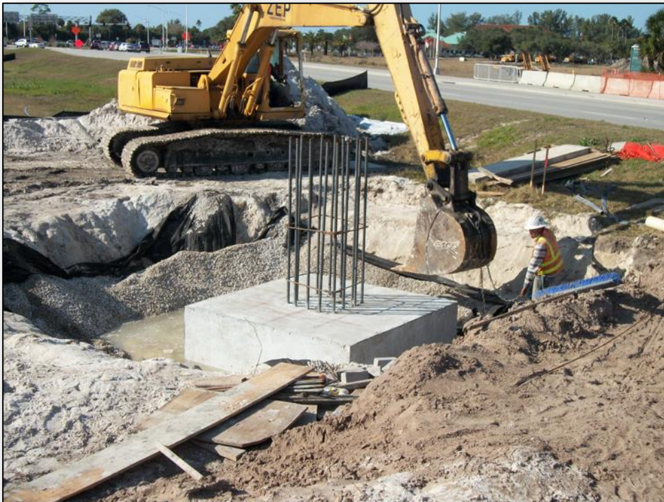
Center tower construction on US 41 in District One.
