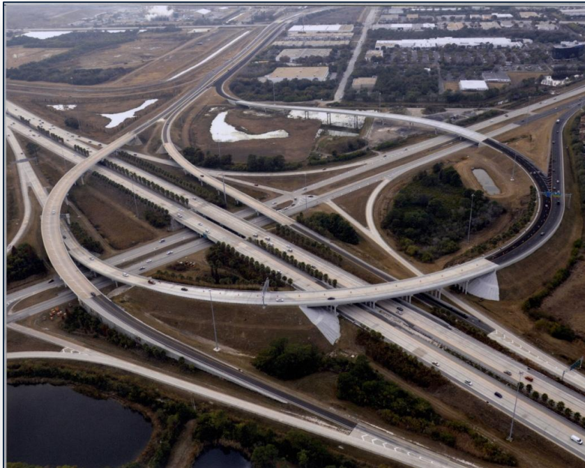
New ramp from Northbound I-275 to 118 th Avenue in Tampa.
