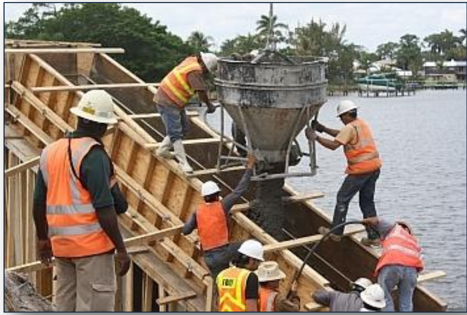
Tequesta Bridge Concrete pour.
