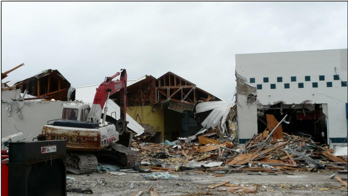
Turnpike Plaza demolition.
