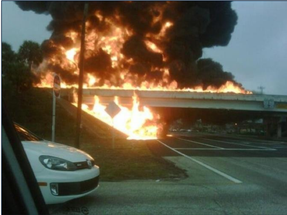
State Road 528 going up in flames after an accident.
