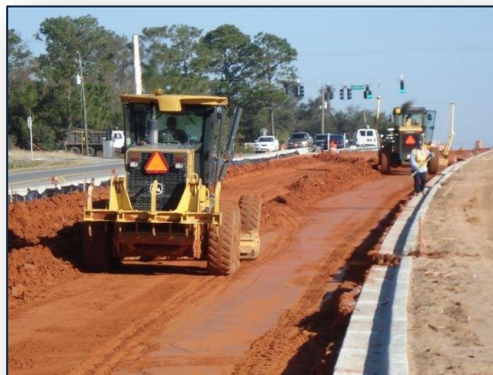
State Road 281 widening project in Santa Rosa County.
