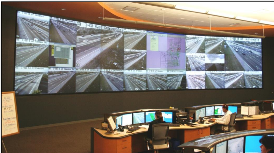
Broward County Traffic Management Center video wall.
