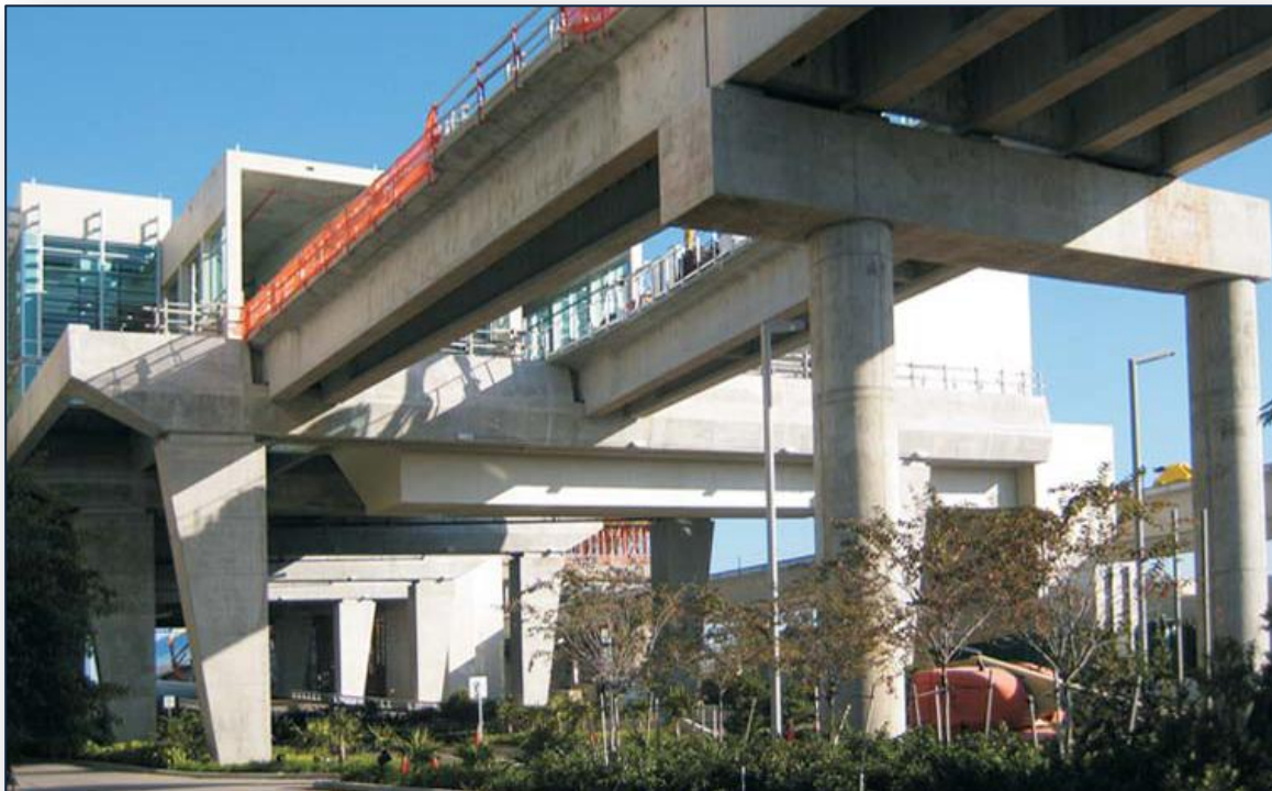
Miami Intermodal Center Construction: MIC/MIA Guideway.
