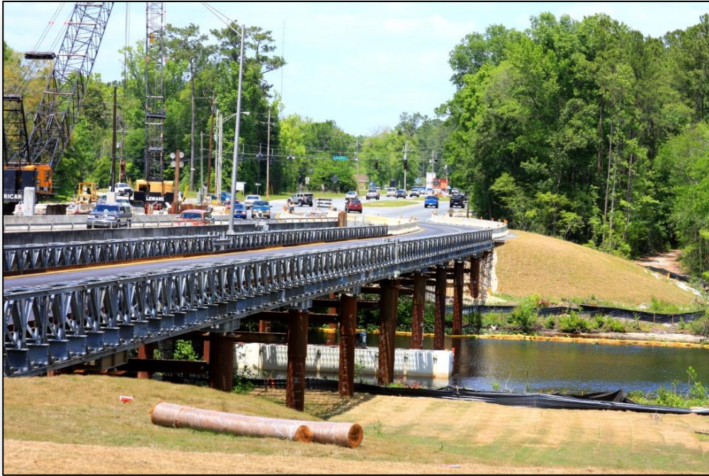
State Road 21, Black Creek Bridge reconstruction.
