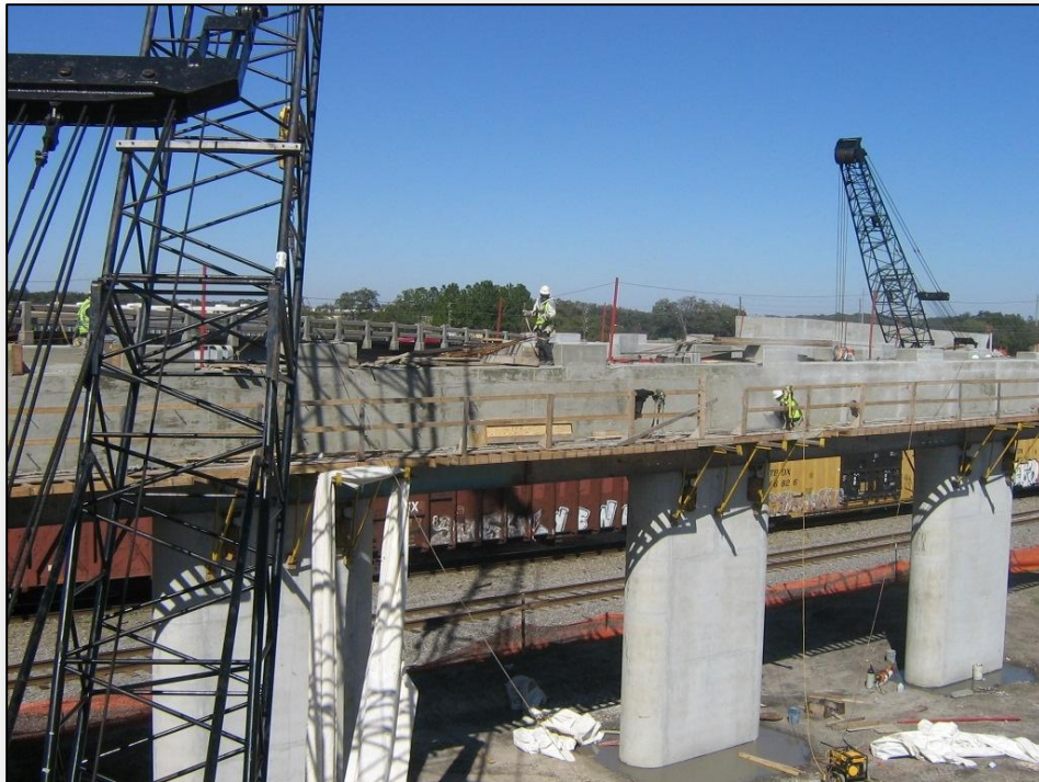
Construction on Pier 2 bridge support on SR 35.
