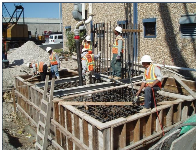
Work on NW 25 th Street in Miami.
