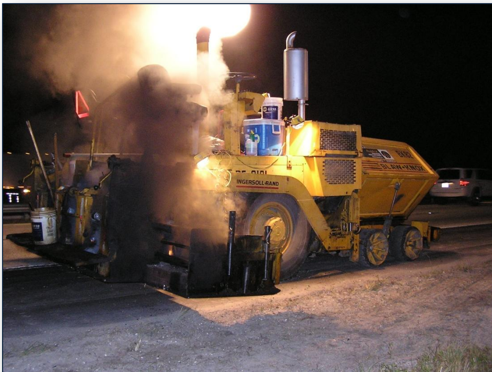
Night work on the IROX (Interstate 75) project in District One.
