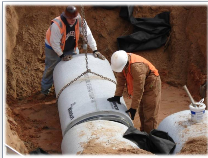
Work on SR 281 (Avalon Boulevard) in District Three.
