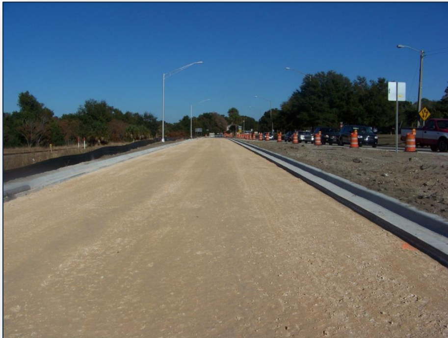
US 17-92 Construction on southbound lanes northeast of new Pomelo Extension.
