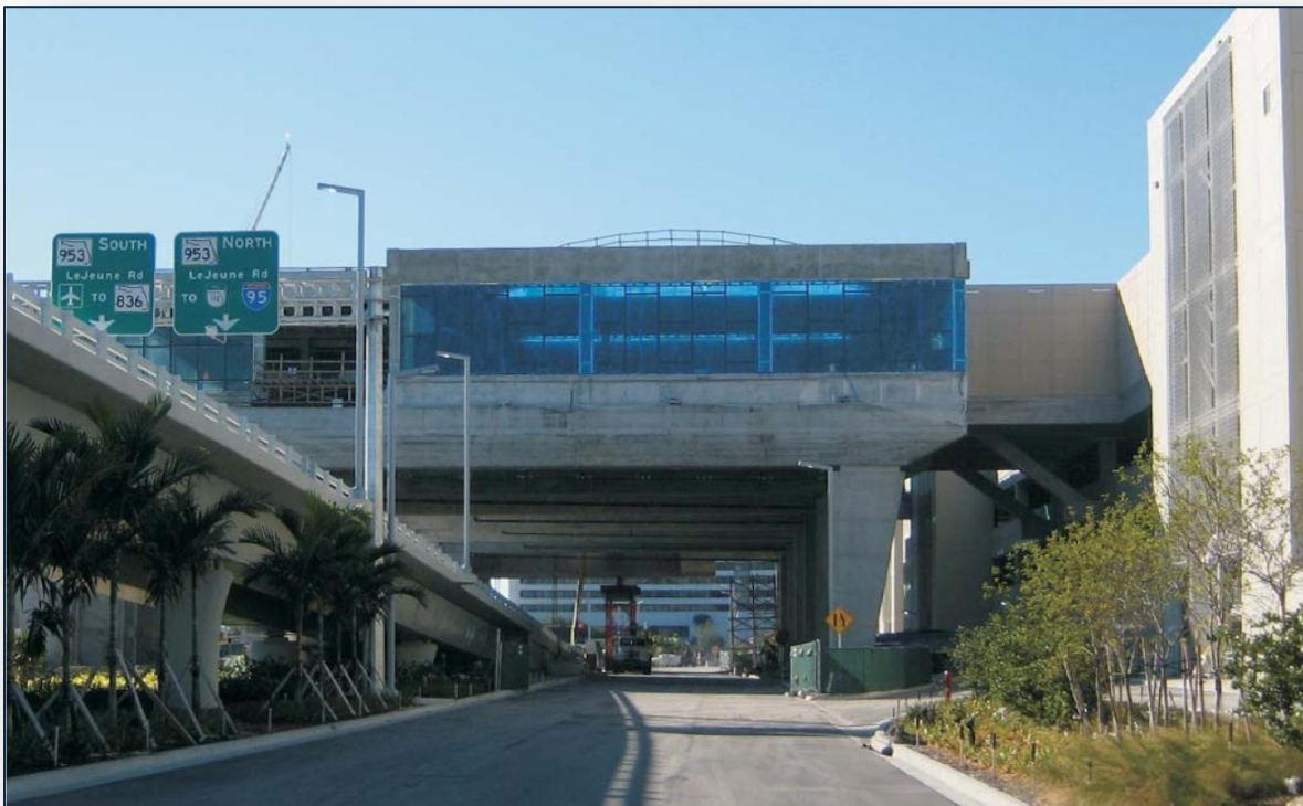
Progress being made on the Miami Intermodal Center.
