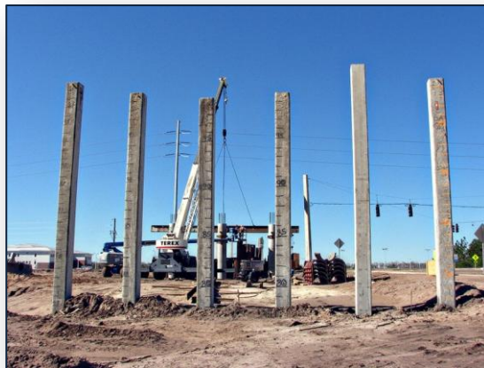
New overpass on SR 23 in Clay County.
