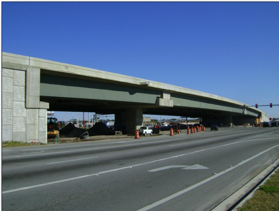
State Road 50 Flyover at SR 436 in Orlando.
