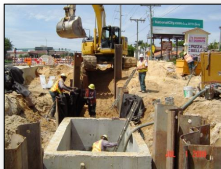
U.S. 1 drainage improvement project.
