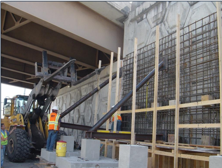
Widening Interstate 95 in Palm Beach County.
