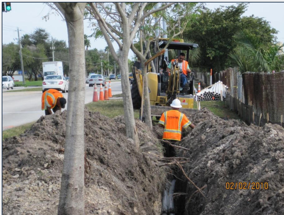
Some of the Palmetto Expressway improvements in Miami.
