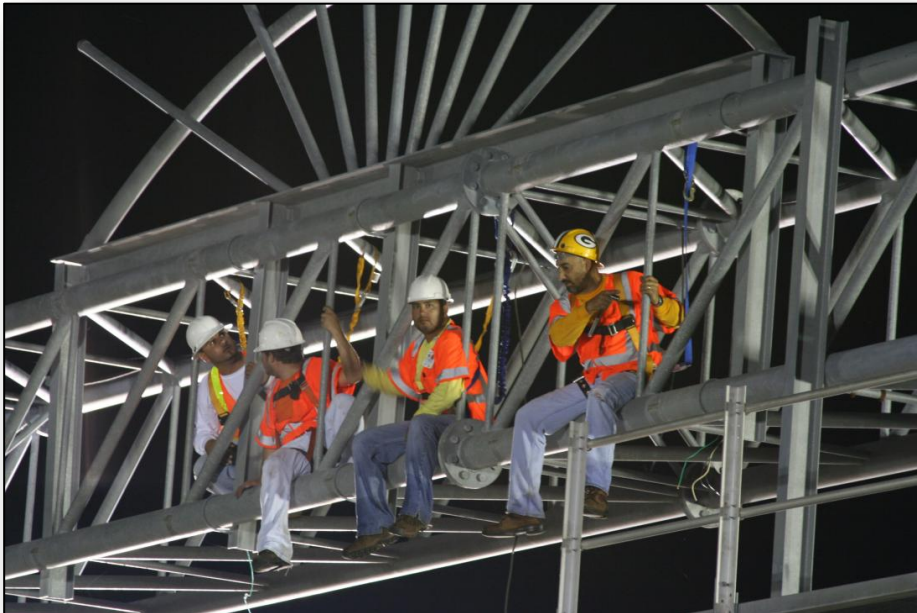
Installing a Dynamic Message Sign in District Four.
