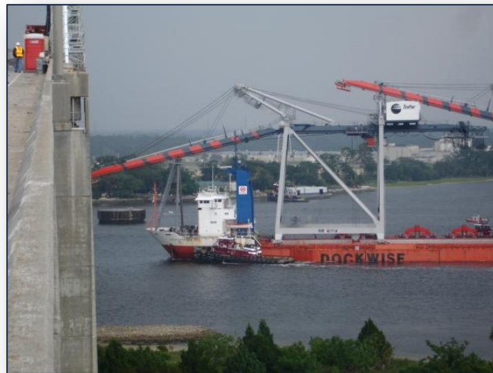
Dames Point Bridge inspection.
