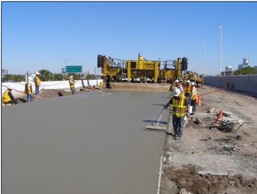
Concrete paving on Interstate 275 east of Armenia Drive in Tampa.
