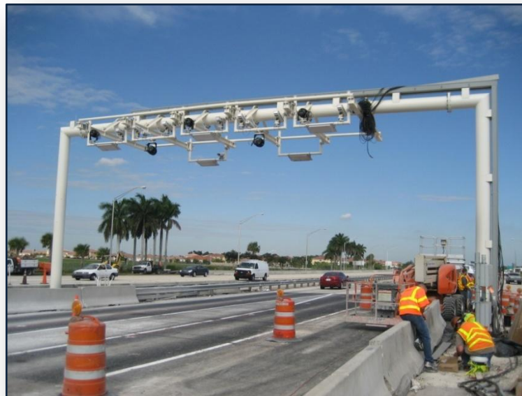
Homestead Open Road Tolling "Lite" construction.
