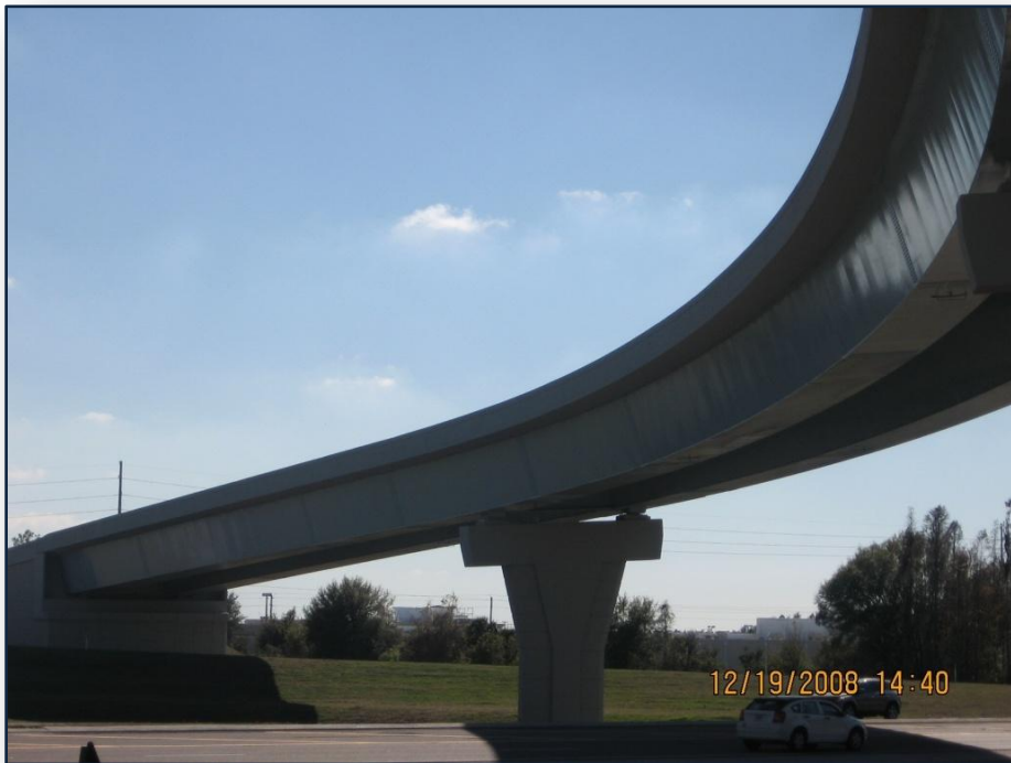
Flyover at Bruce B. Downs Blvd. and Interstate 75 in Tampa.
