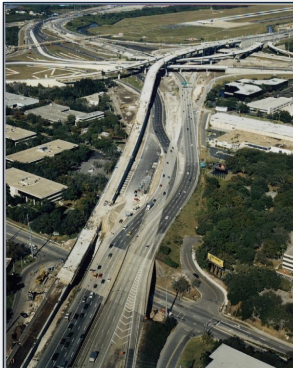
SR 60 looking north from Cypress Street towards Tampa International Airport.
