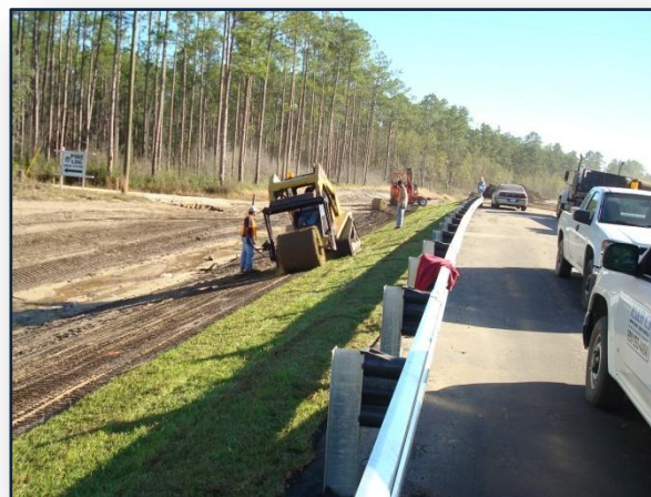
Slope work on SR 79 in Bay County.
