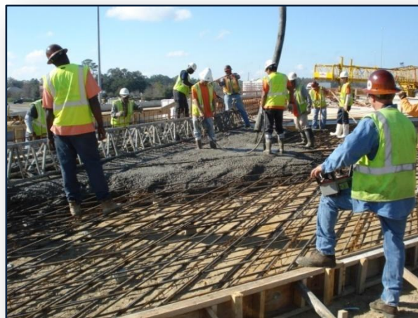
Bridge work on Interstate 10 in Leon County.
