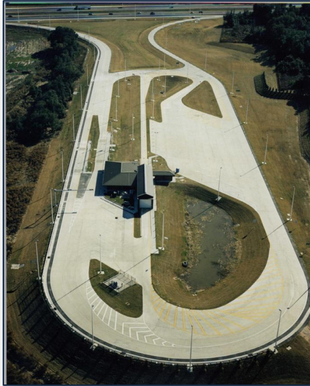
Looking south at the new I-4 Weigh-in-Motion Station, located between Tampa and Plant City.
