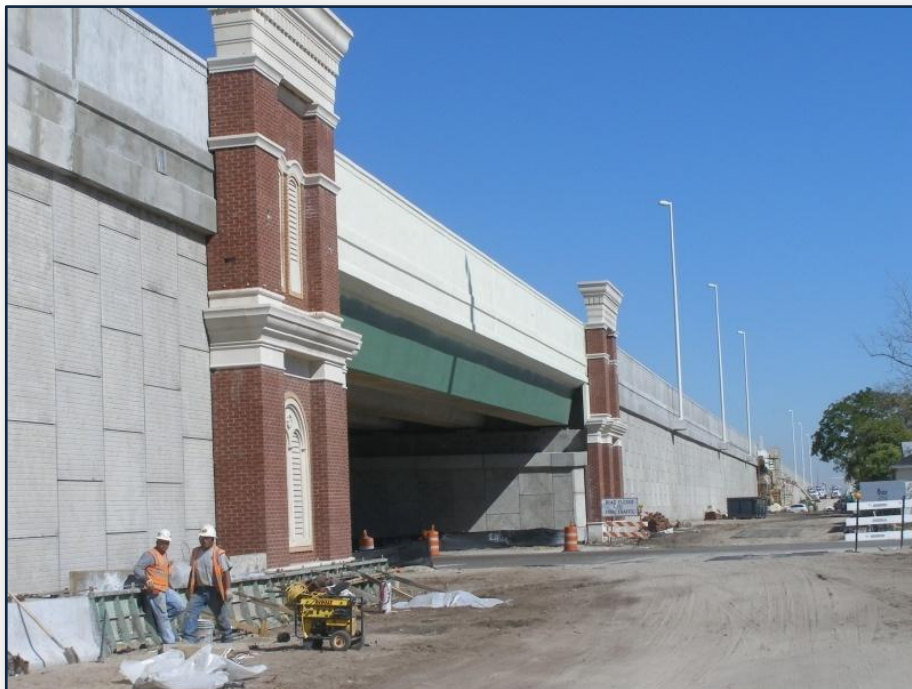
Art Deco bridge construction at Armenia Drive in Tampa.
