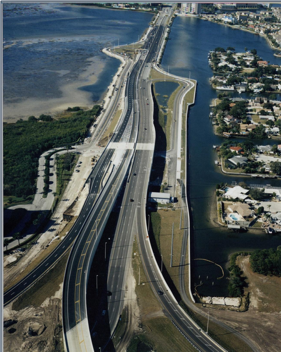
Looking west at SR 60 between Memorial Highway and Rocky Point Drive.
