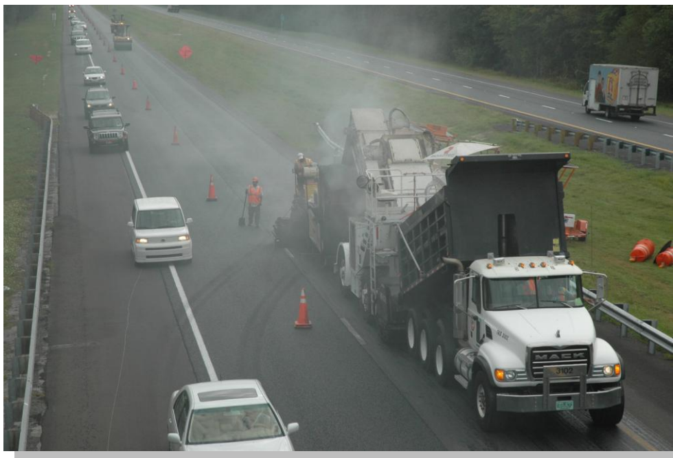
Resurfacing work on Interstate 10.
