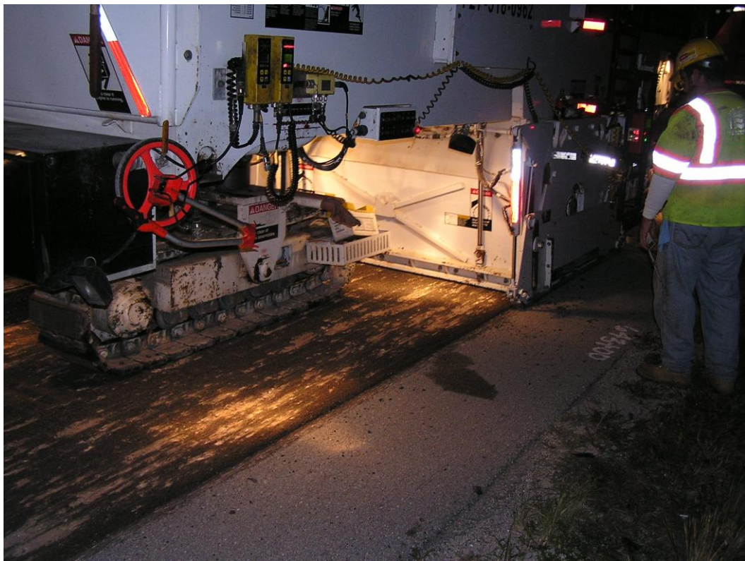
Nighttime milling work on Interstate 75 in Southwest Florida.
