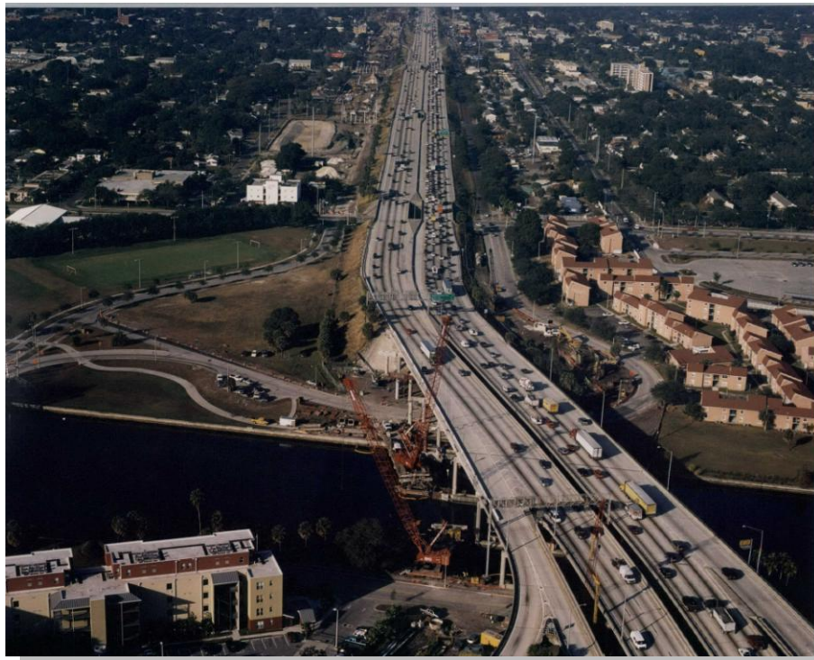
Interstate 275 construction over the Hillsborough River.
