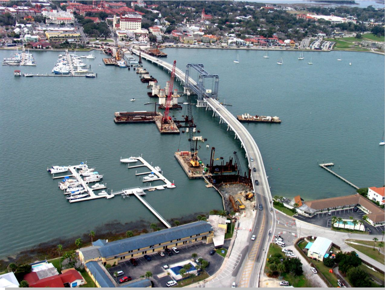
Bridge of Lions rehabilitation project in St. Augustine.
