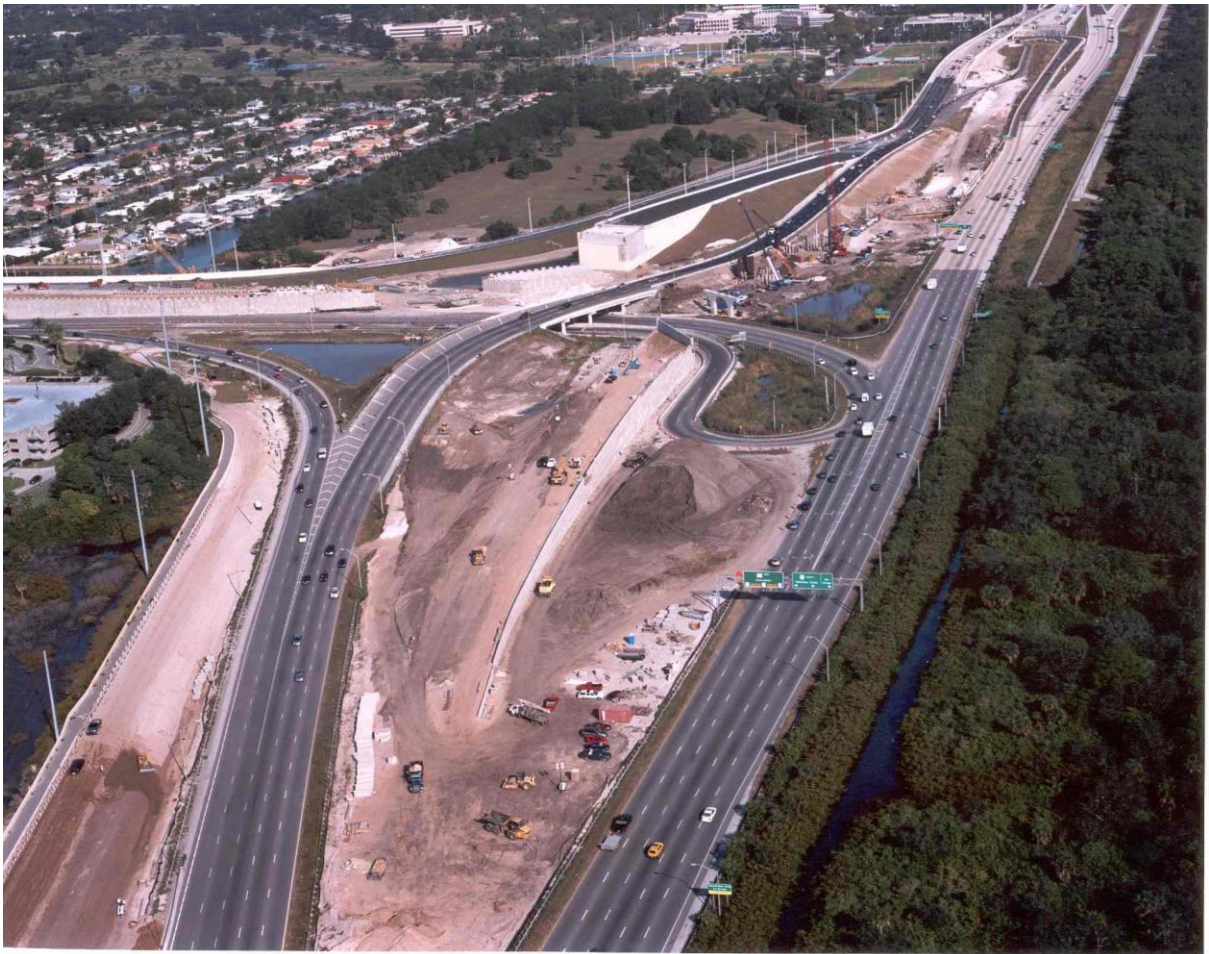
Tampa International Airport interchange construction.
