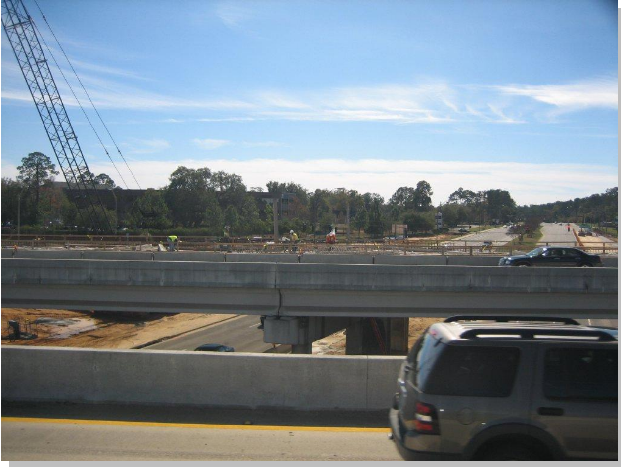
Interstate 10 reconstruction in Tallahassee.
