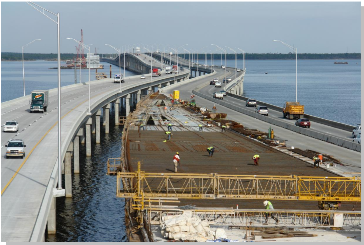
Escambia Bay Bridge replacement.
