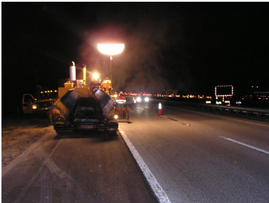
Nighttime shoulder work on Interstate 75 in Southwest Florida.
