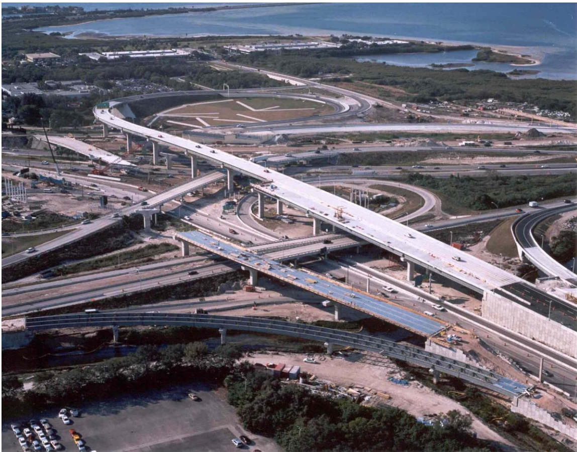
Tampa International Airport Interchange improvements.
