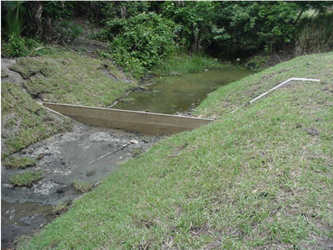
Figure 2. Parkland Wetland weir
