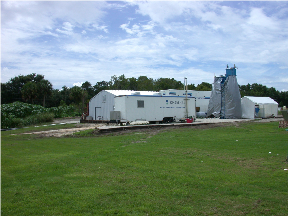
Figure 1. Pilot facility at City of Sanford water reclamation facility
