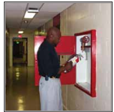
North Region Fire Protection Specialist Eric Bryant Inspects a Fire Extinguisher at a University Residential Housing Unit
