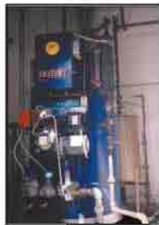
Heating Boiler Installed in Hotel
