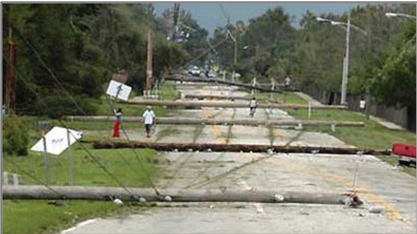
Hazardous Conditions Orange County
