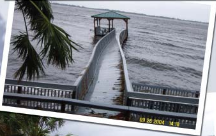
Damage from Hurricane Jeanne - Shoreside Park, Town of Palm Shores
