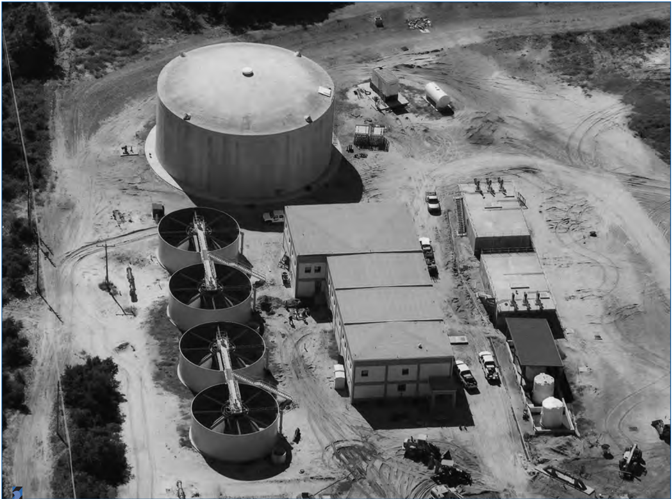
City of Port St. Joe water treatment plant
