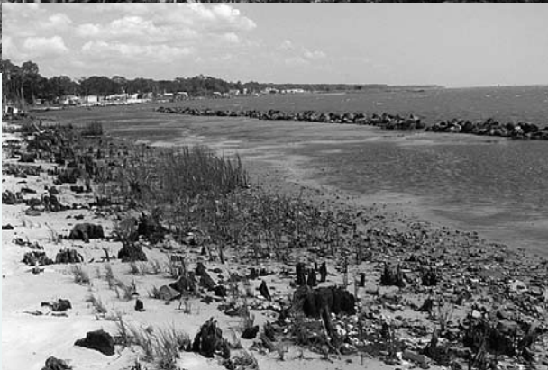
Cat Point, an Apalachicola Bay breakwater and salt marsh restoration site, is located in Eastpoint, Franklin County. Through this project, 0.8 acres of shoreline were restored to mitigate for a 0.3-acre impact to seagrass beds in Apalachicola Bay with the replacement of the St. George Island Bridge. The project will be used to educate the general public about alternatives to shoreline hardening techniques that result in the loss of aquatic and upland habitat. The site was planted with nearly ten thousand smooth cordgrass ( Spartina alterniflora ) tubelings as well as upland buffer species such as saltmeadow cordgrass ( Spartina patens ), muhly grass ( Muhlenbergia capillaris ) and saltbush ( Baccharis hamlimiflora ).
