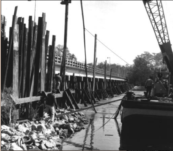
Dead Lakes Dam removed.
