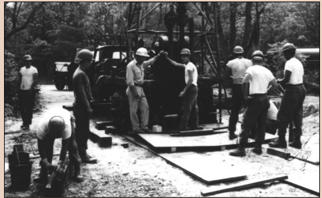
Well drilling in the northwest.
