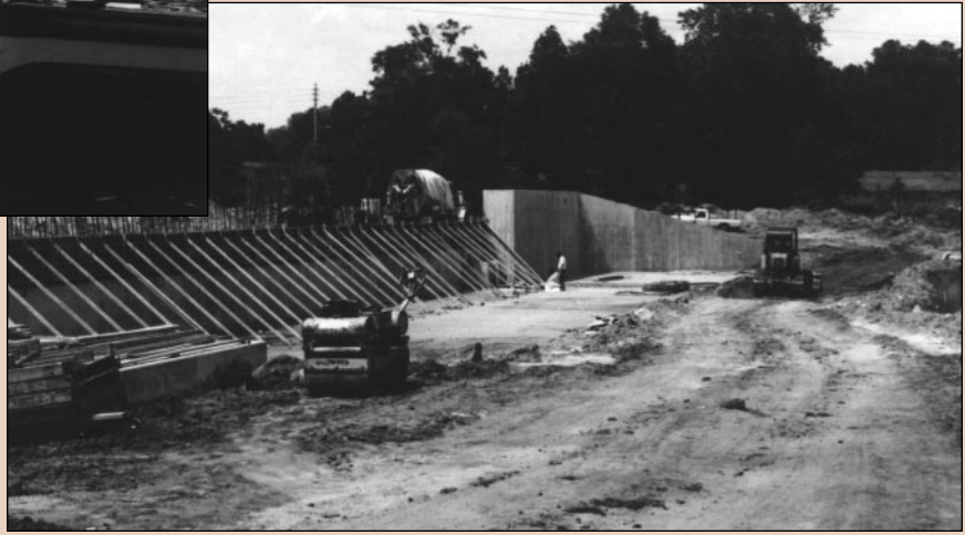
Lake Jackson Meginniss Arm Stormwater Treatment Facility constructed.
