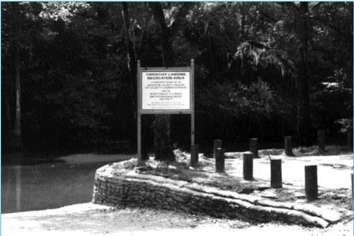
Christoff Landing was a cooperative project of the District and Jackson County.
