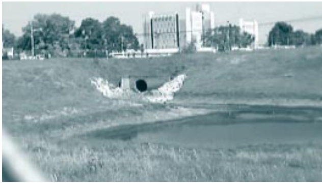
Alum Injection Stormwater Project
