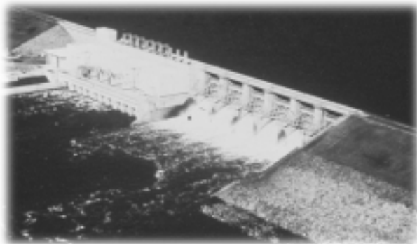
Jim Woodruff Lock and Dam at Lake Seminole.
