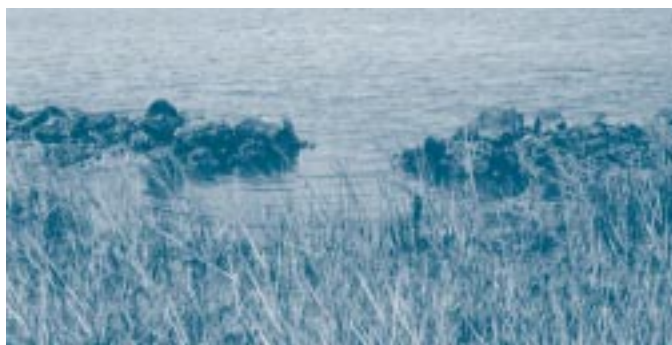
A constructed breakwater at St. George Island.
