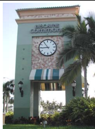
Biscayne Commons is built on a Brownfield site in Miami-Dade County
