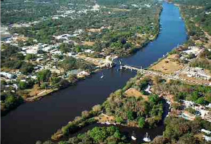
LaBelle, FL in Hendry County at the Caloosahatchee River Bridge looking west.
