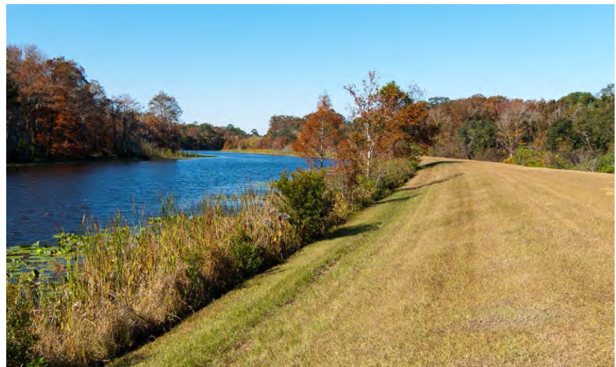
A levee system at Sunnyhill Restoration Area helps manage water on the property.
