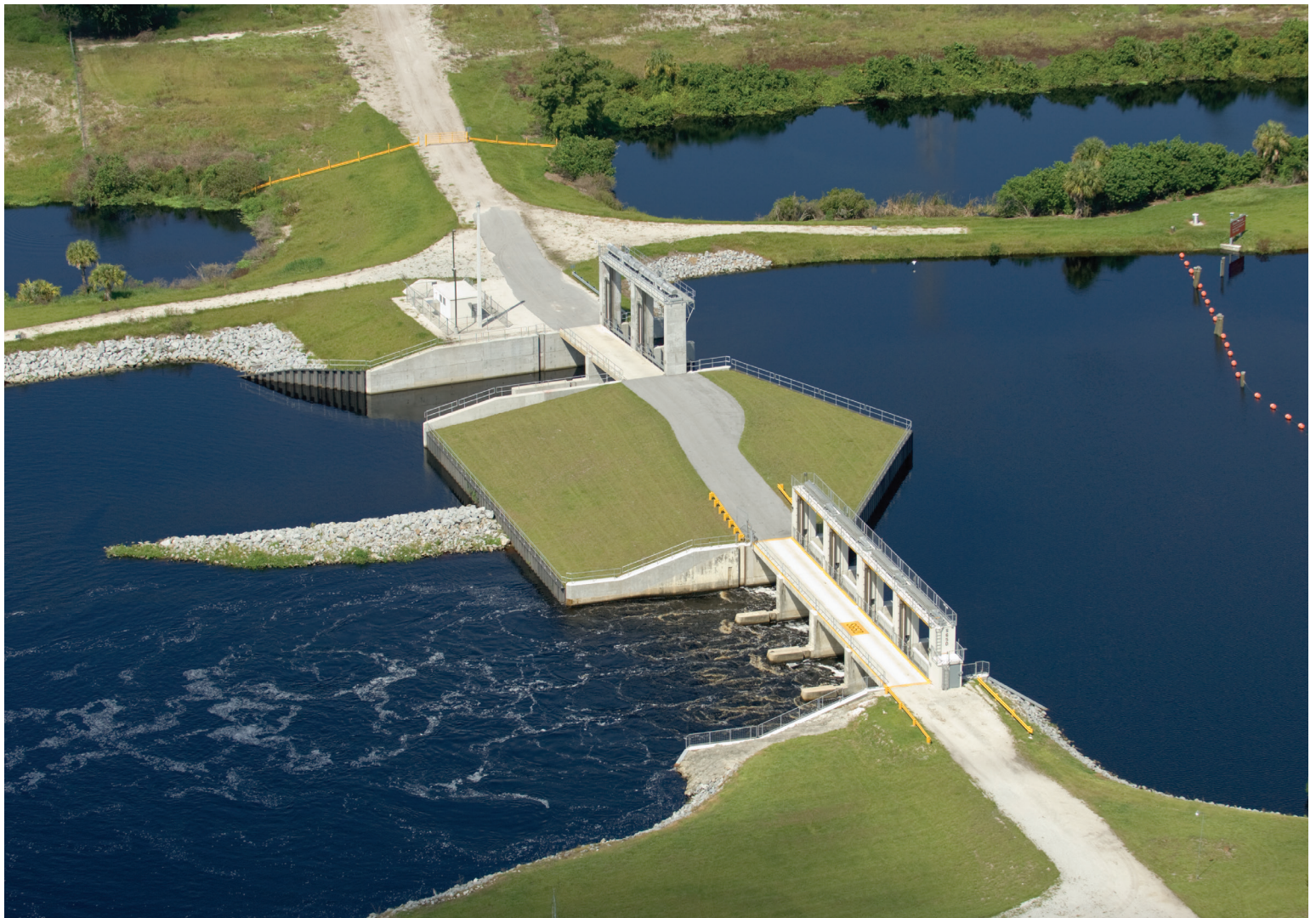
Kissimmee River Structure Gate S-65D
