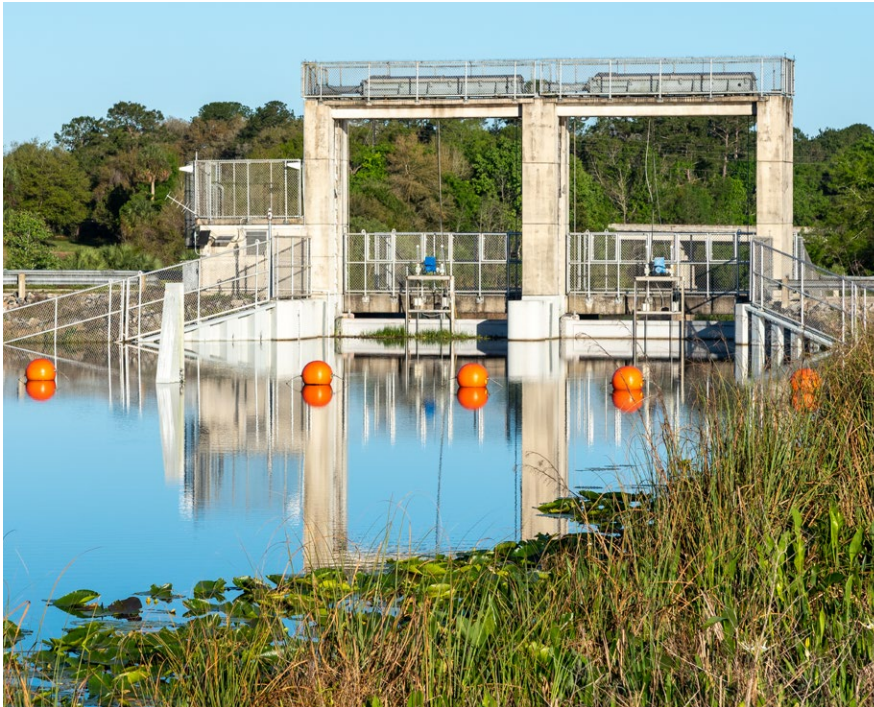
The Moss Bluff structure helps regulate water levels.
