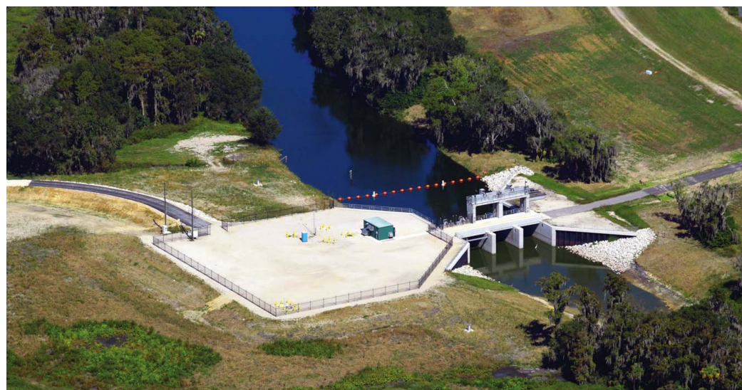
Construction of the P-11 structure replacement was completed in April 2013.
