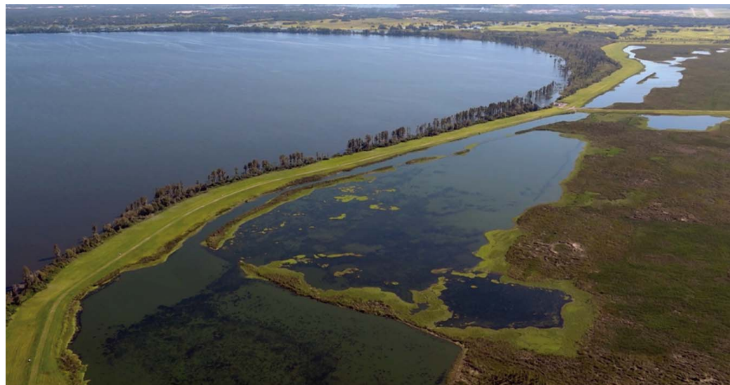
Lake Hancock Outfall Treatment System.
