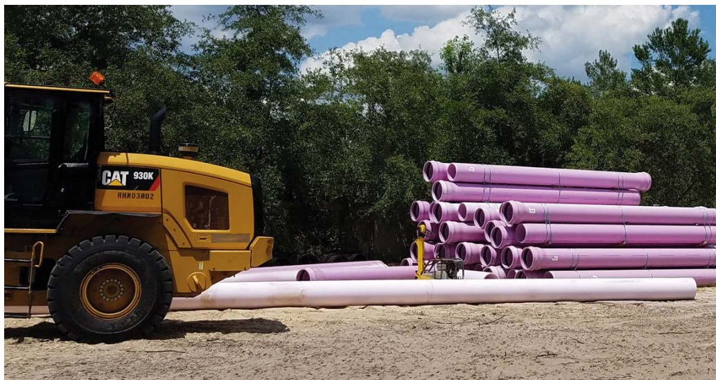
Reuse pipeline construction site.
