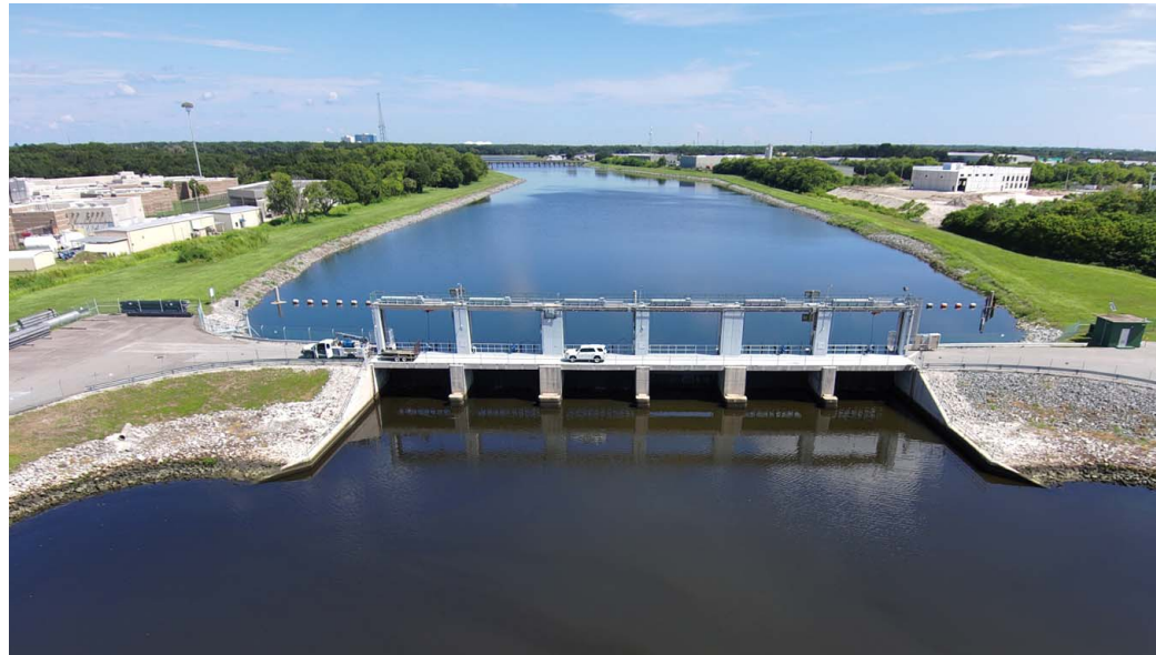
Tampa Bypass Canal.
