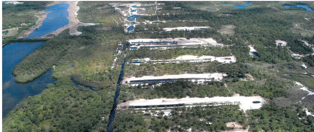
Newly created freshwater wetlands at Coral Creek, Phase 2 in Charlotte County.
