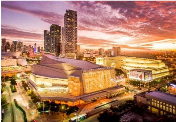
Adrienne Arsht Center for the Performing Arts of Miami-Dade County
