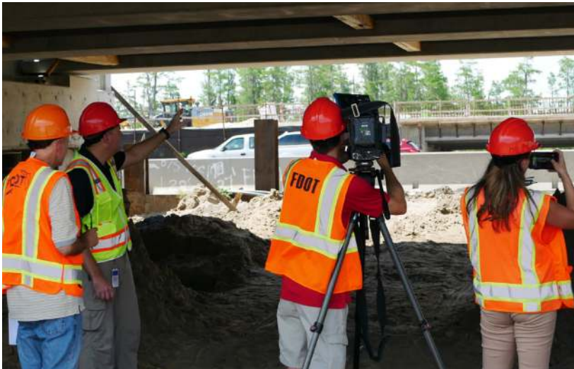
FDOT District 1 Drainage Design Engineer, Brent Setchell, is seen leading one of several press events at the I-4/S.R. 557 Wildlife Crossing currently under construction in Polk County.
