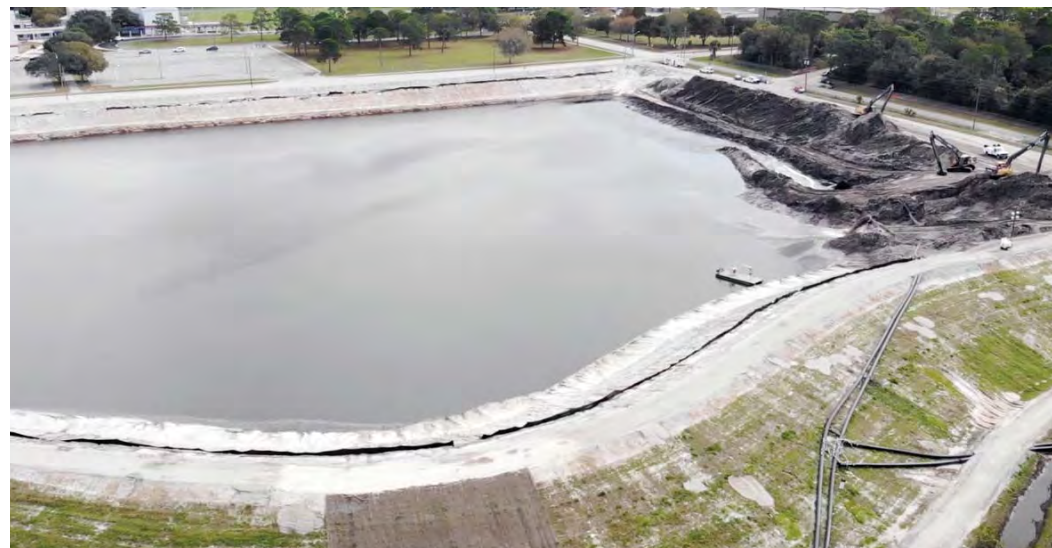
Lake Seminole dredge material management area.
