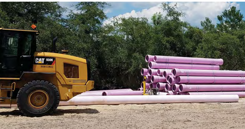
Reuse pipeline construction site.
