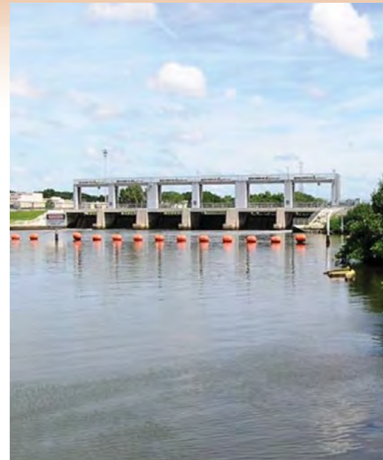
The District's S-160 Structure on the Tampa Bypass Canal in Hillsborough County.
