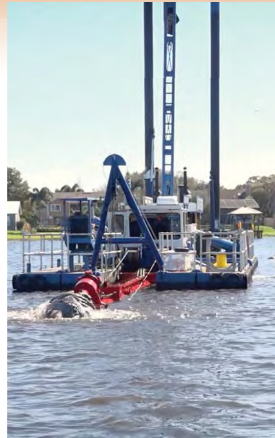
Dredging on Lake Seminole in Pinellas County.
