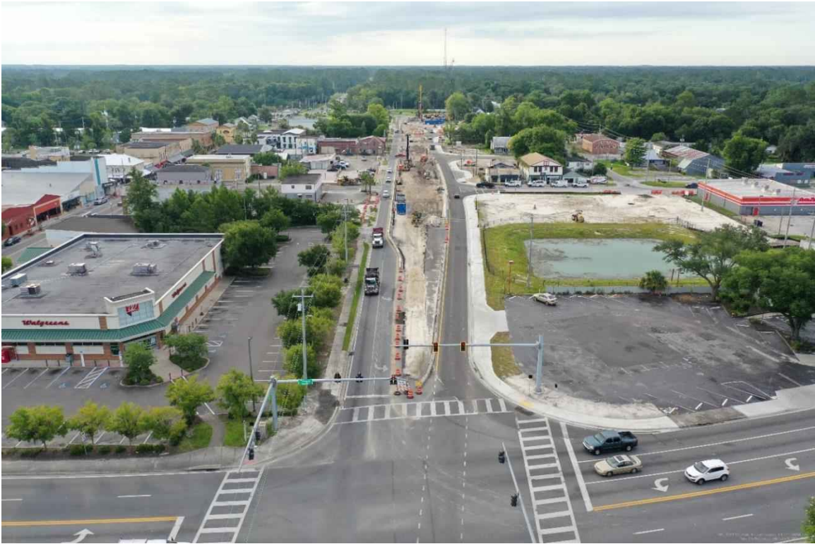
Starke Road Overpass Project (District 2)
