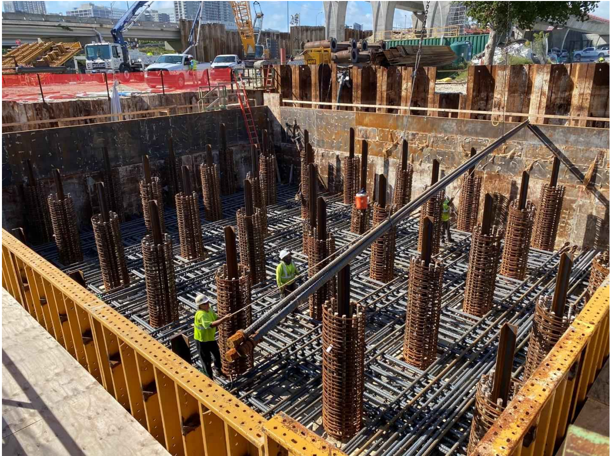
SR 836/I-395/I-95 Design Build Project (District 6)
