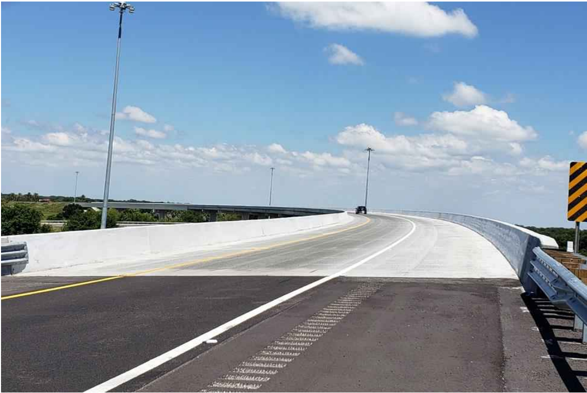
I-275 at I-75 Northbound Overpass Deck Replacement (District 1)
