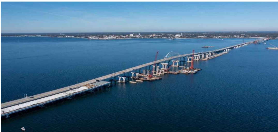
Pensacola Bay Bridge (District 3)
