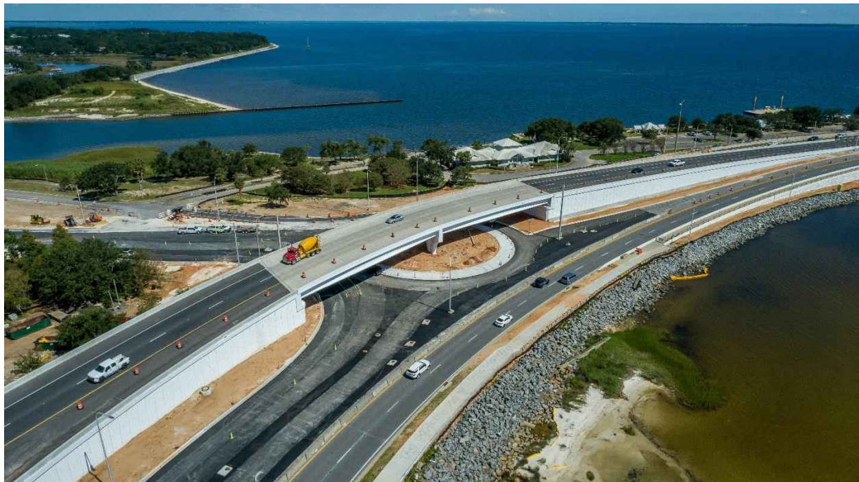
17 th Avenue Interchange Construction (District 3)
