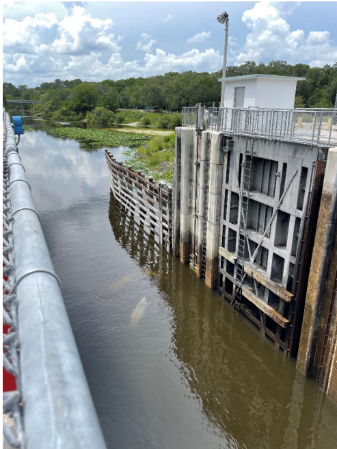
Photo of Moss Bluff Lock in Marion County taken at the 2023 Annual Manatee Water Control Structure Working Group Meeting
