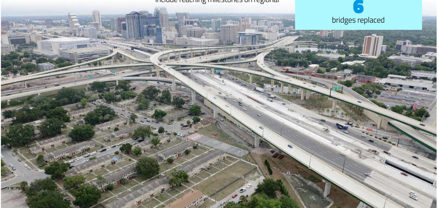
I-4 and S.R. 408 Interchange on the I-4 Ultimate project
