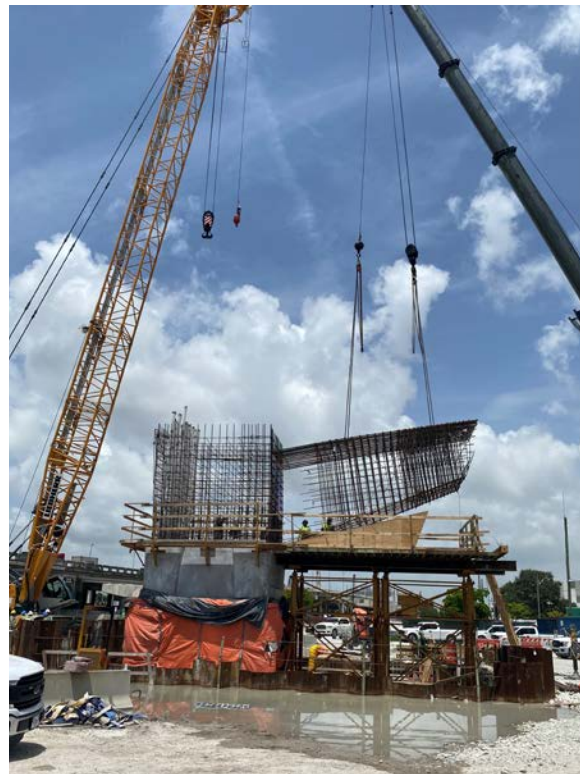
I-395 Pier Construction
