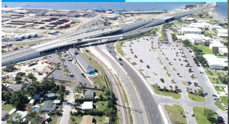
23rd Street Flyover
