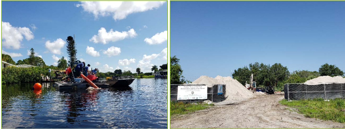
Photos of Warm Mineral Springs restoration project, Sarasota County.
