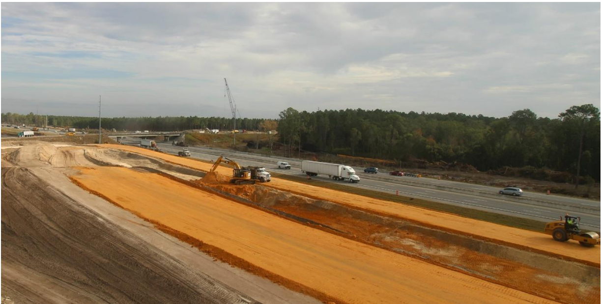
New Interchange at I-75 and Overpass Road – District 7
