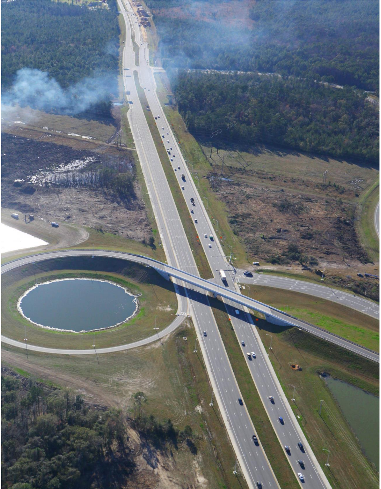
First Coast Expressway – District 2
