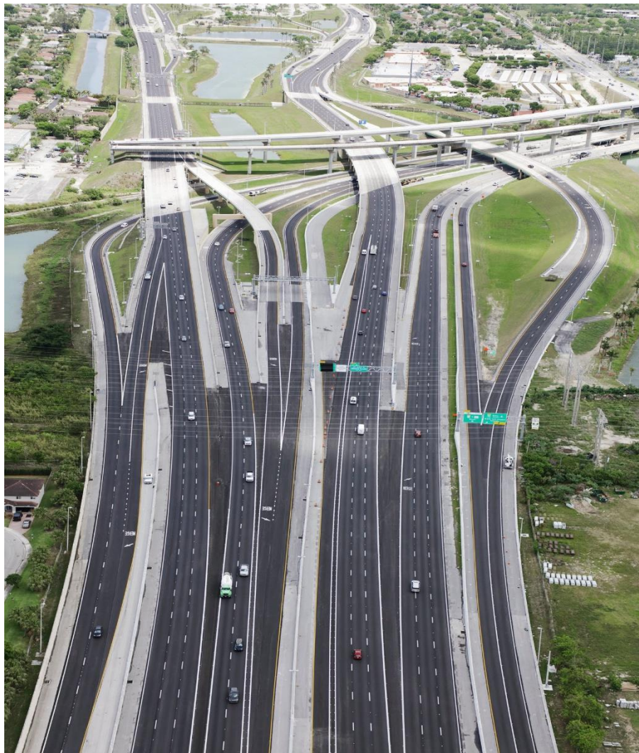
HEFT Widening – Florida Turnpike
