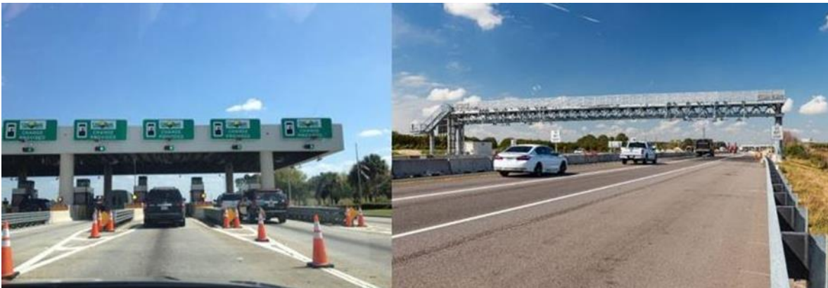
Northern Coin Conversion – Florida Turnpike
