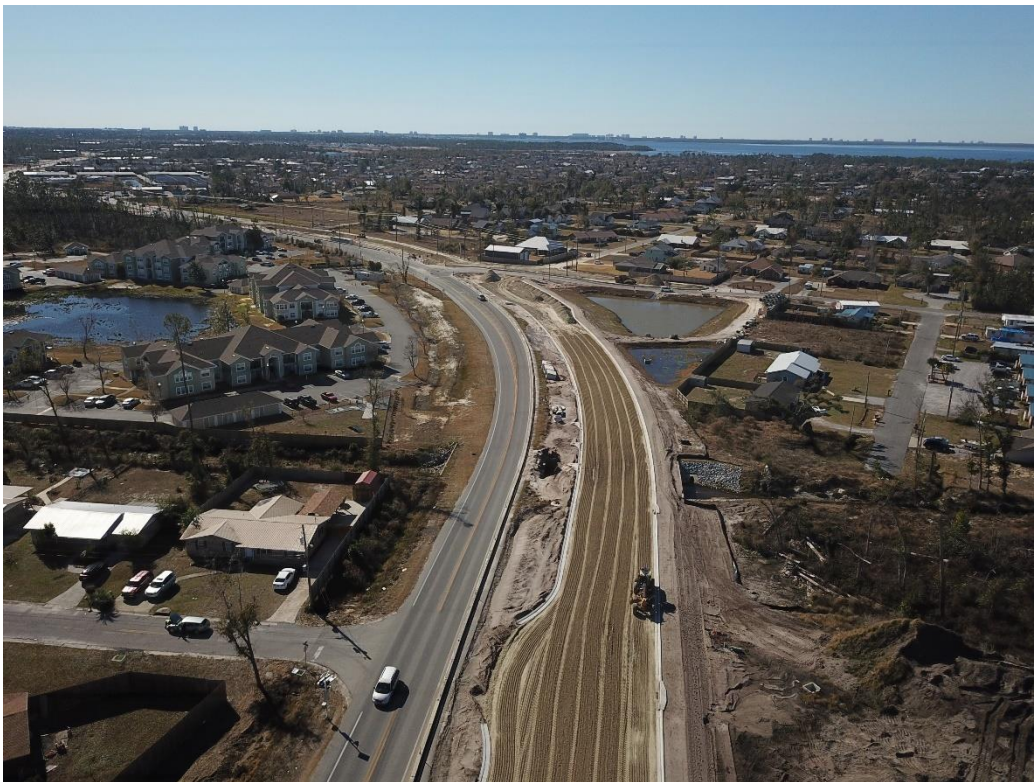
State Road 390 Widening – District 3
