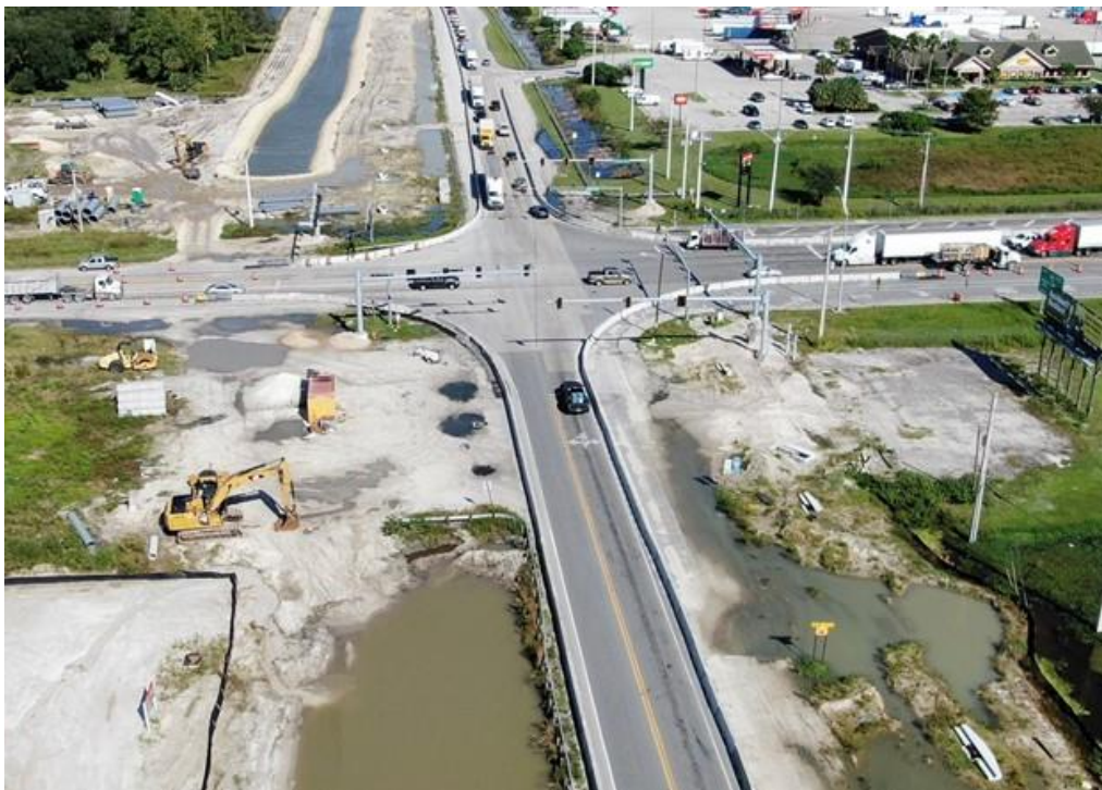
Kings Highway Widening – District 4
