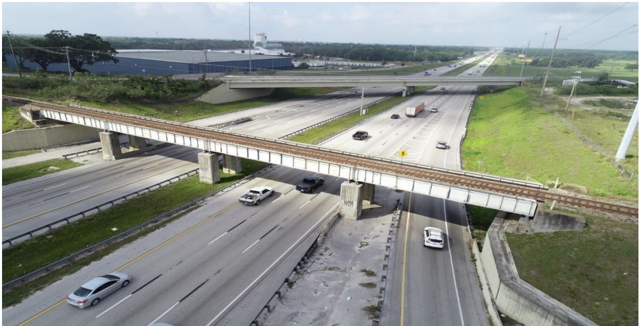
I-4 at CSX Railroad Bridge Replacement – District 1
