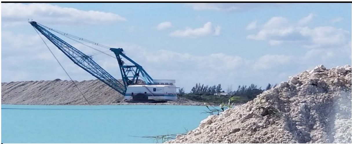
Excavated above ground limerock pile
