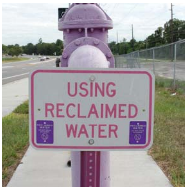
Reclaimed water line.
