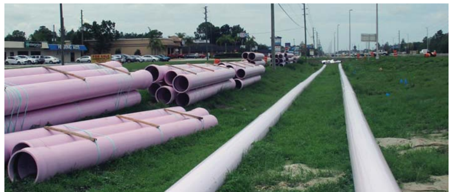
Reclaimed water transmission line construction project on U.S. 19 in Hernando County.
