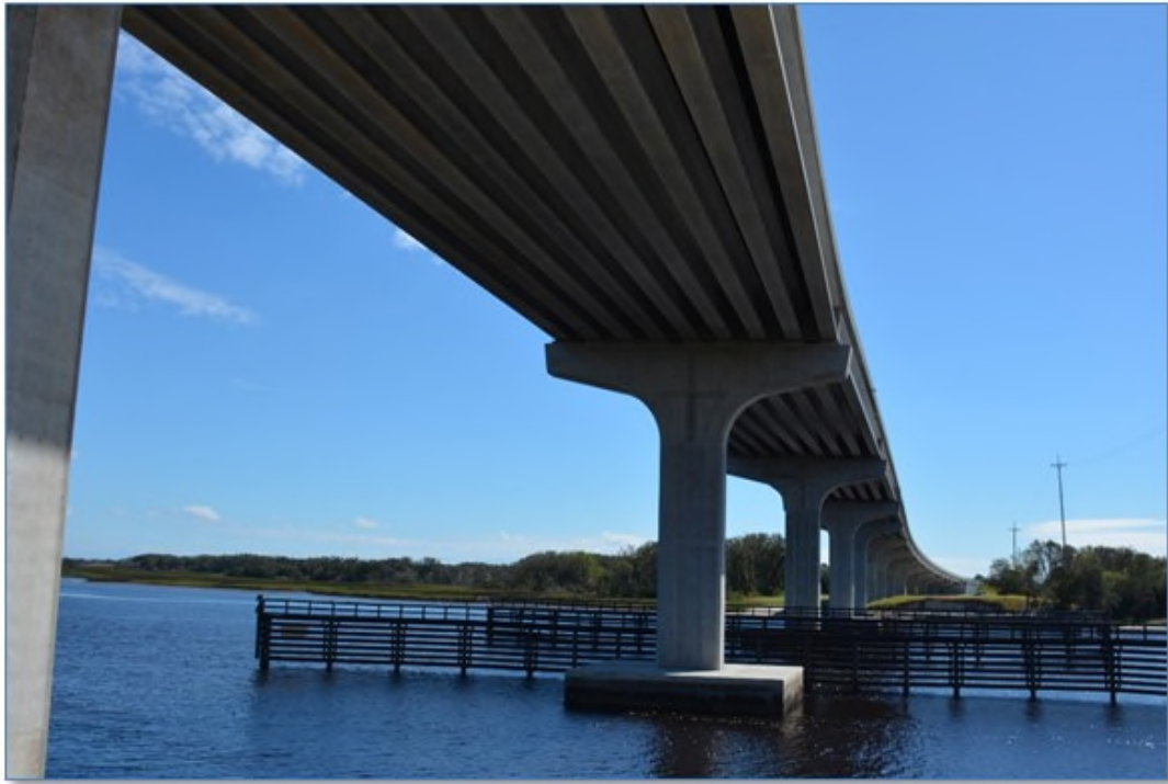
Sisters Creek Bridge Replacement – District 2
