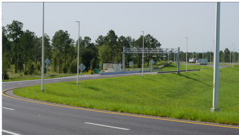
Completed Turnpike/Hancock Road Interchange at Milepost 278
