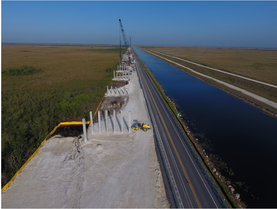
Tamiami Trail Bridge – District 6
