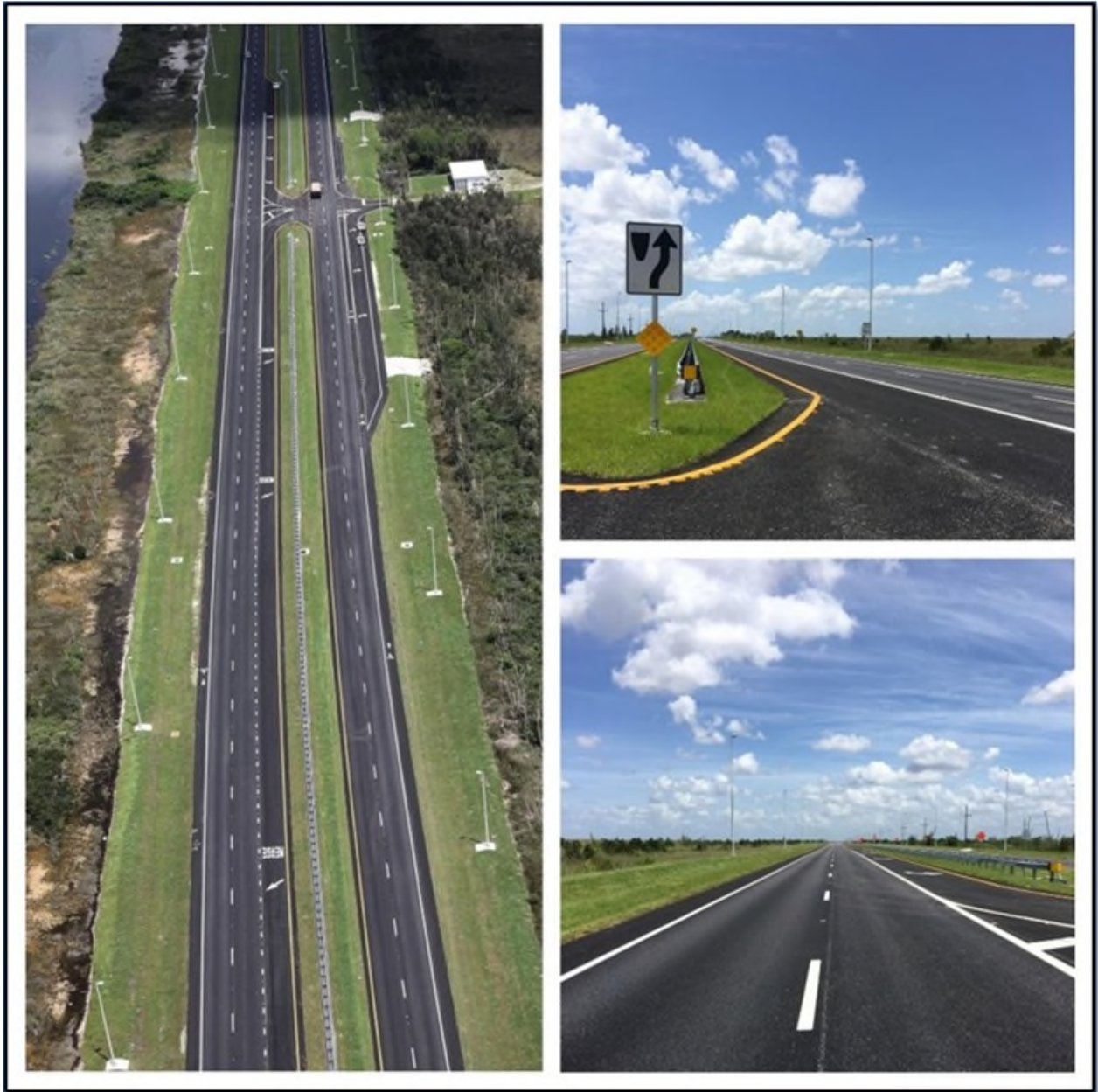
Completed Krome Avenue – District 6
