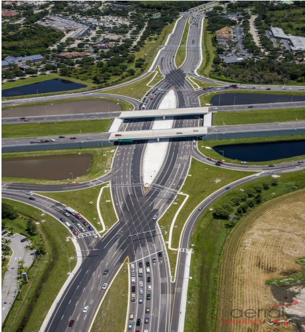
Diverging Diamond Interchange – District 1
