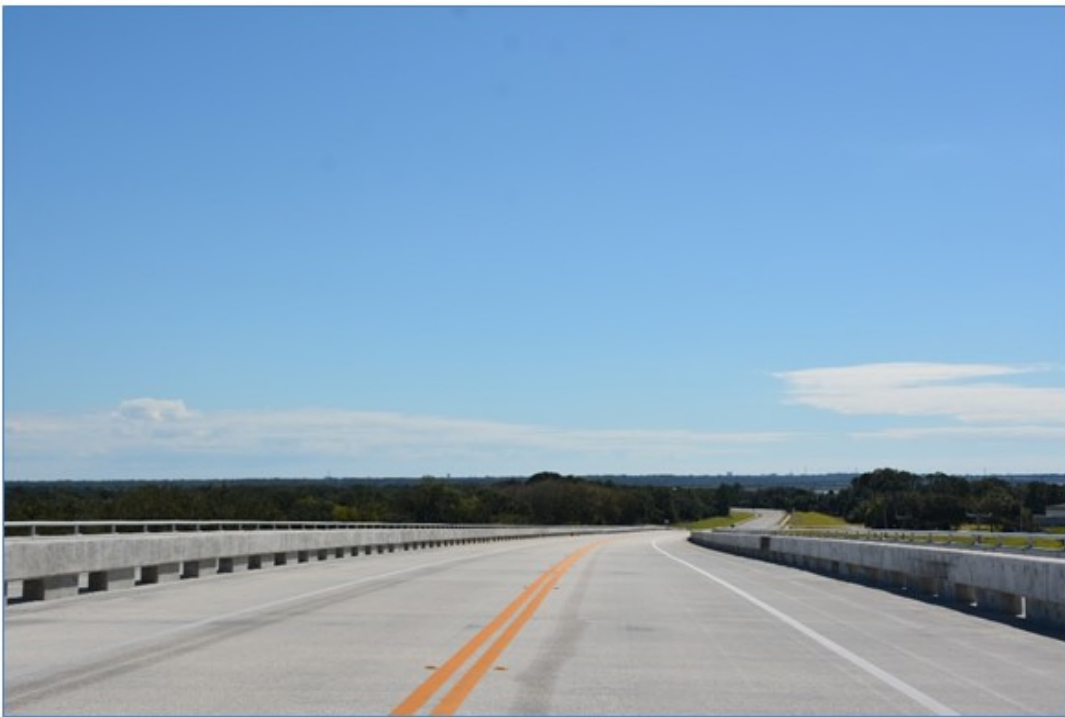
Sisters Creek Bridge Replacement – District 2
