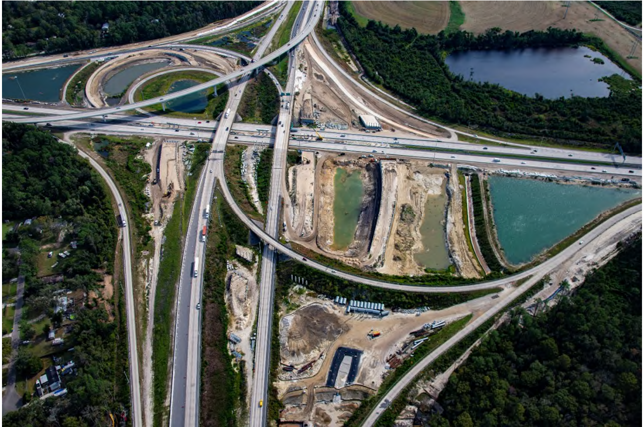
I-95 and I-295N Interchange Reconfiguration
