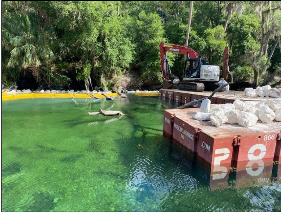
Photo of shoreline stabilization project in Blue Spring Run, Volusia County.
