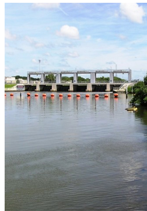
The District's S-160 Structure on the Tampa Bypass Canal in Hillsborough County.
