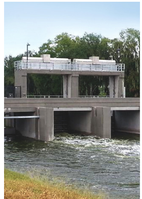
The District's P-11 Water Conservation Structure on Lake Hancock in Polk County.
