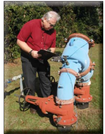
FPSC staff monitors quality-of-service issues such as water pressure and capacity.
