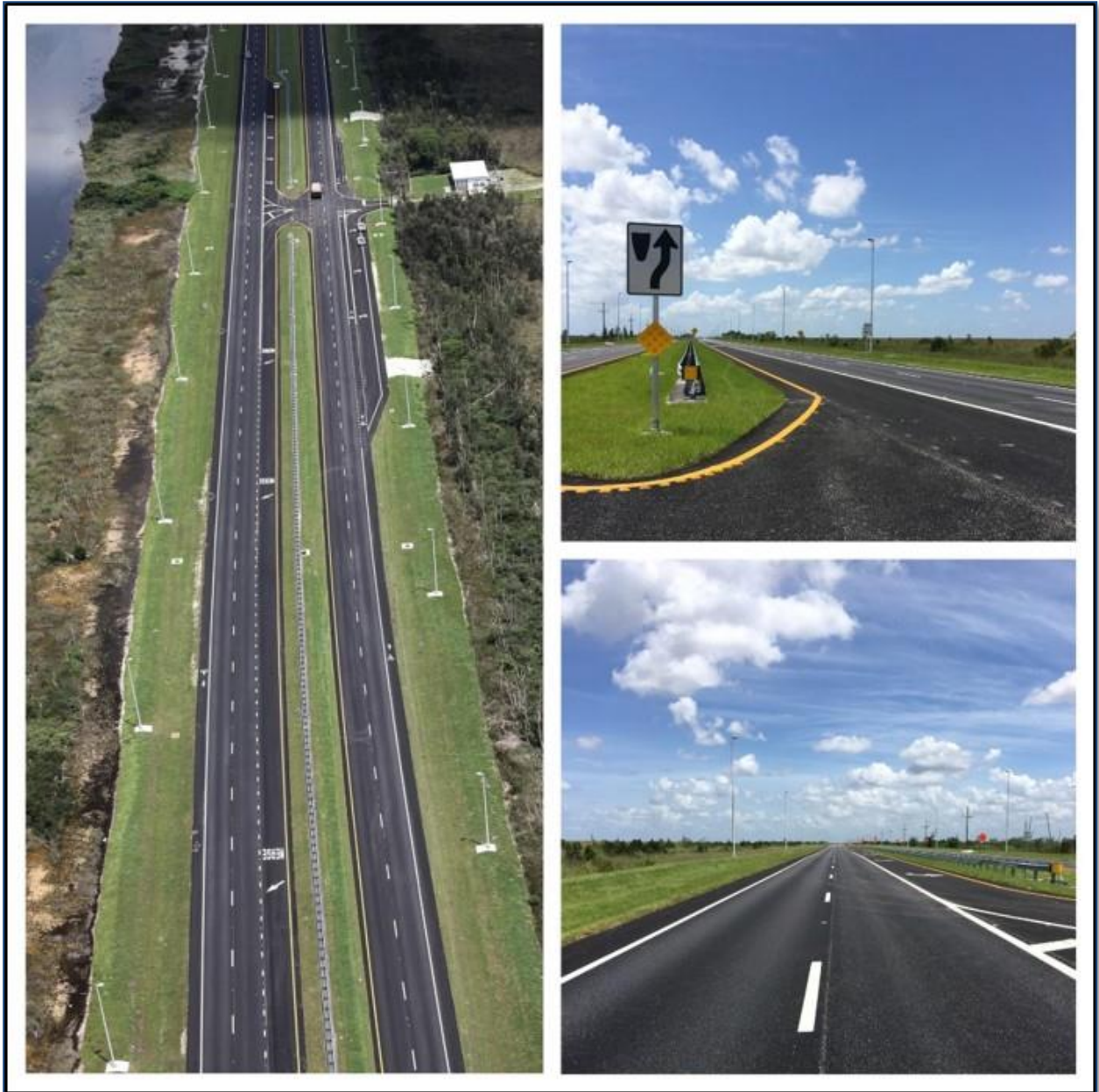
Completed Krome Avenue – District 6
