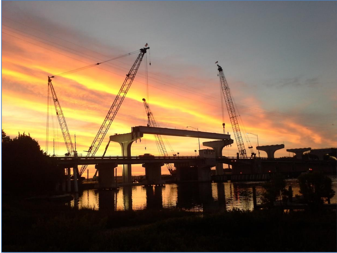
Sisters Creek Bridge Replacement – District 2
