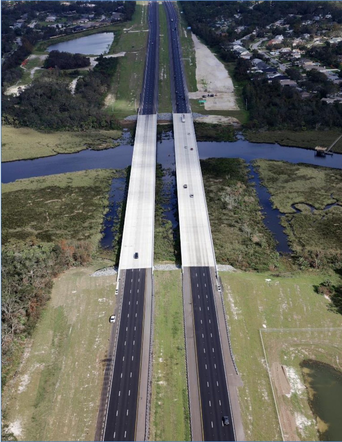
I-95 Widening and System Interchange – District 5
