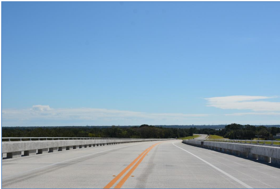
Sisters Creek Bridge Replacement – District 2
