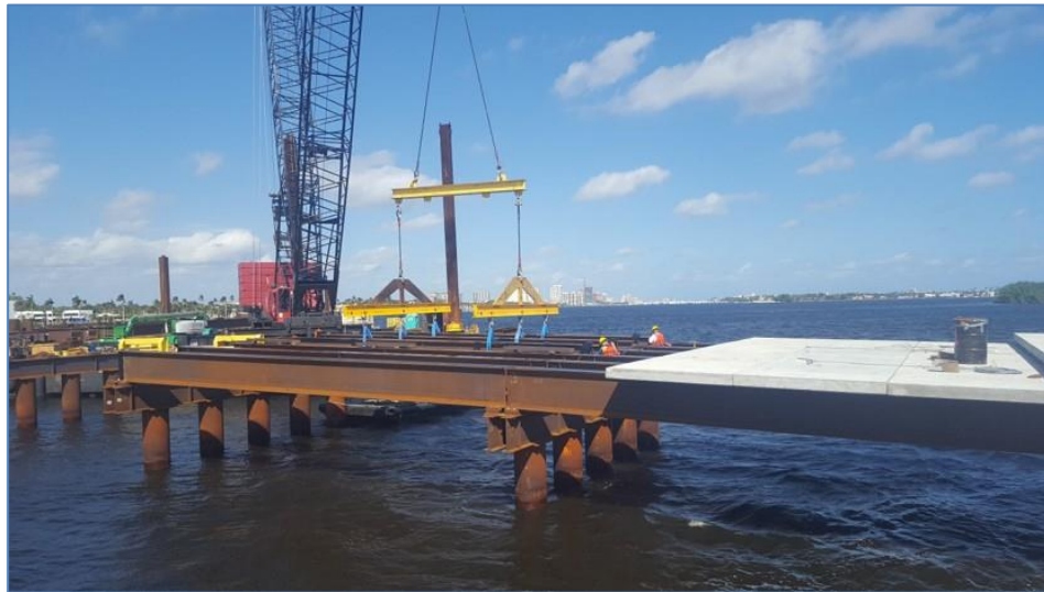
Southern Boulevard Bridge – District 4
