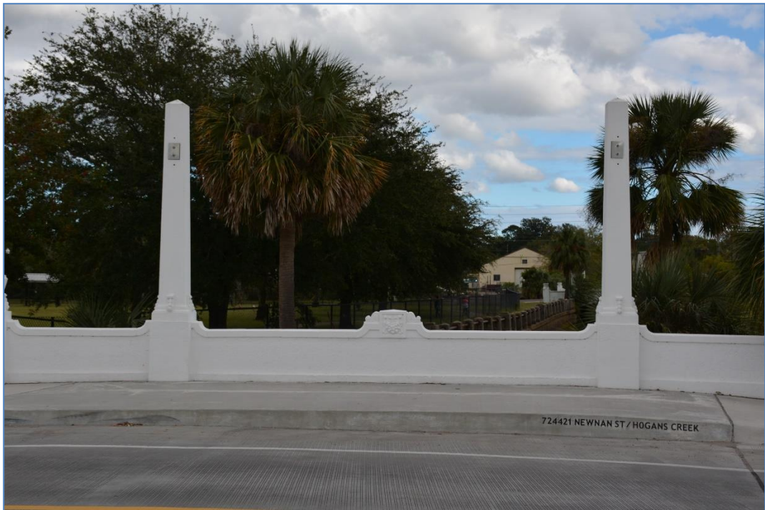
Historical Bridge Repair over Hogan's Creek – District 2
