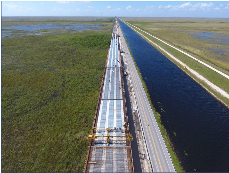
Tamiami Trail Bridge – District 6
