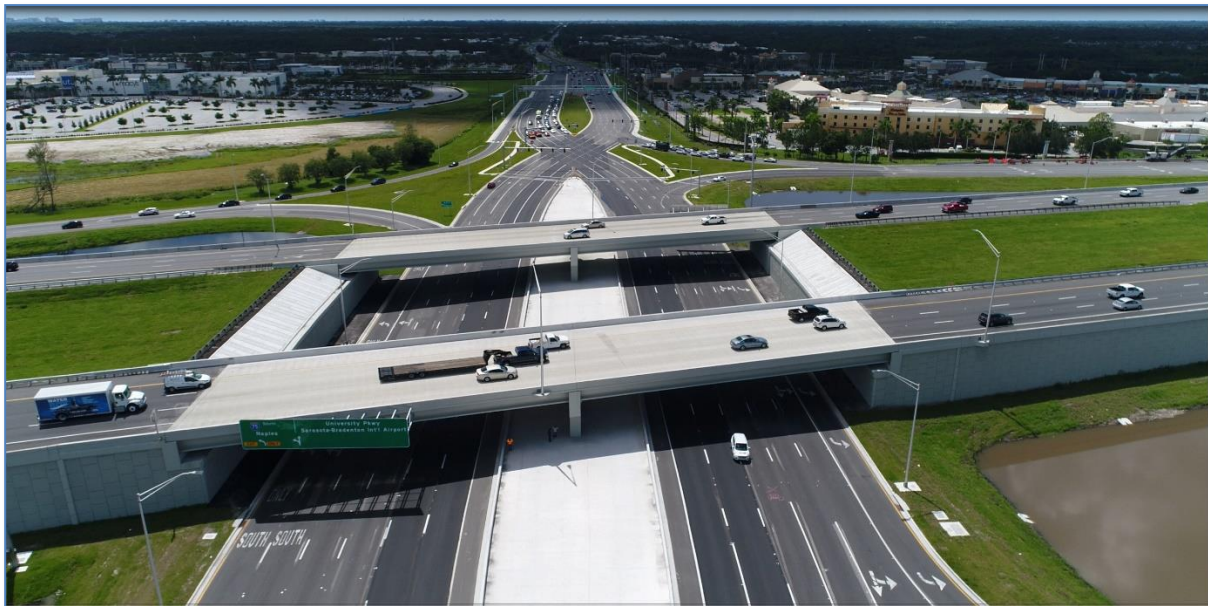
Diverging Diamond Interchange – District 1
