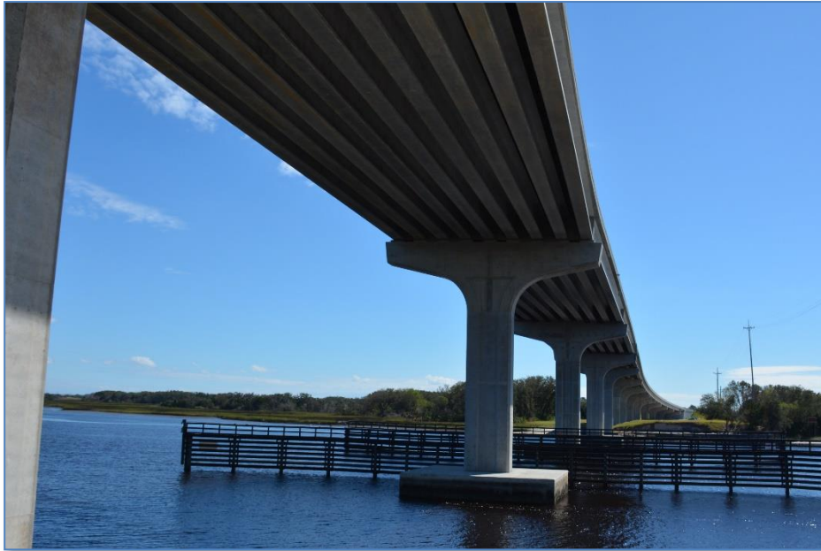
Sisters Creek Bridge Replacement – District 2
