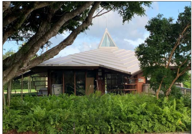
The Visitor Center at the Naples Preserve
