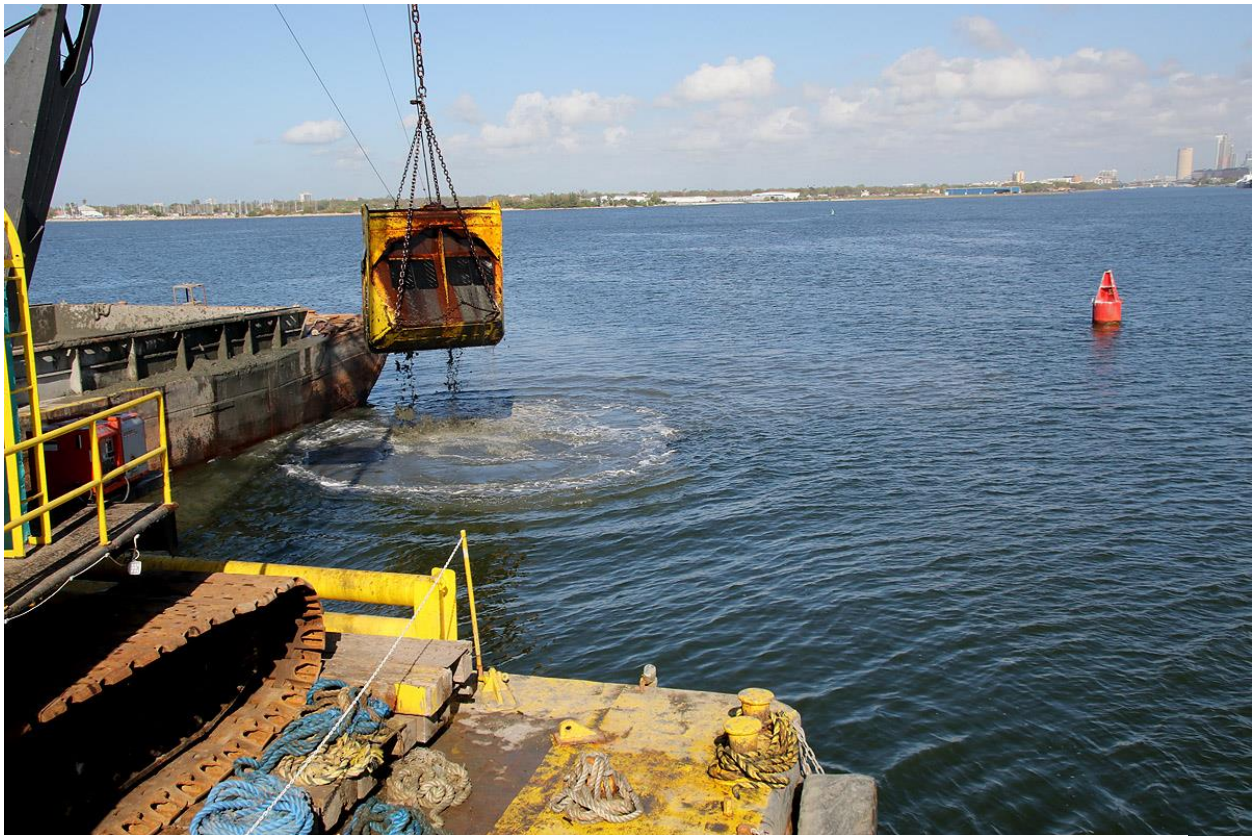
Photo of Clam Shell dredge in Tampa Bay
