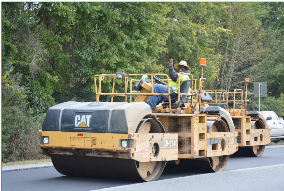
Happy Construction Worker in District Two
