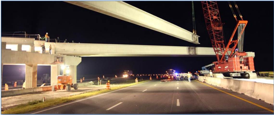
SR 9B Construction in District Two
