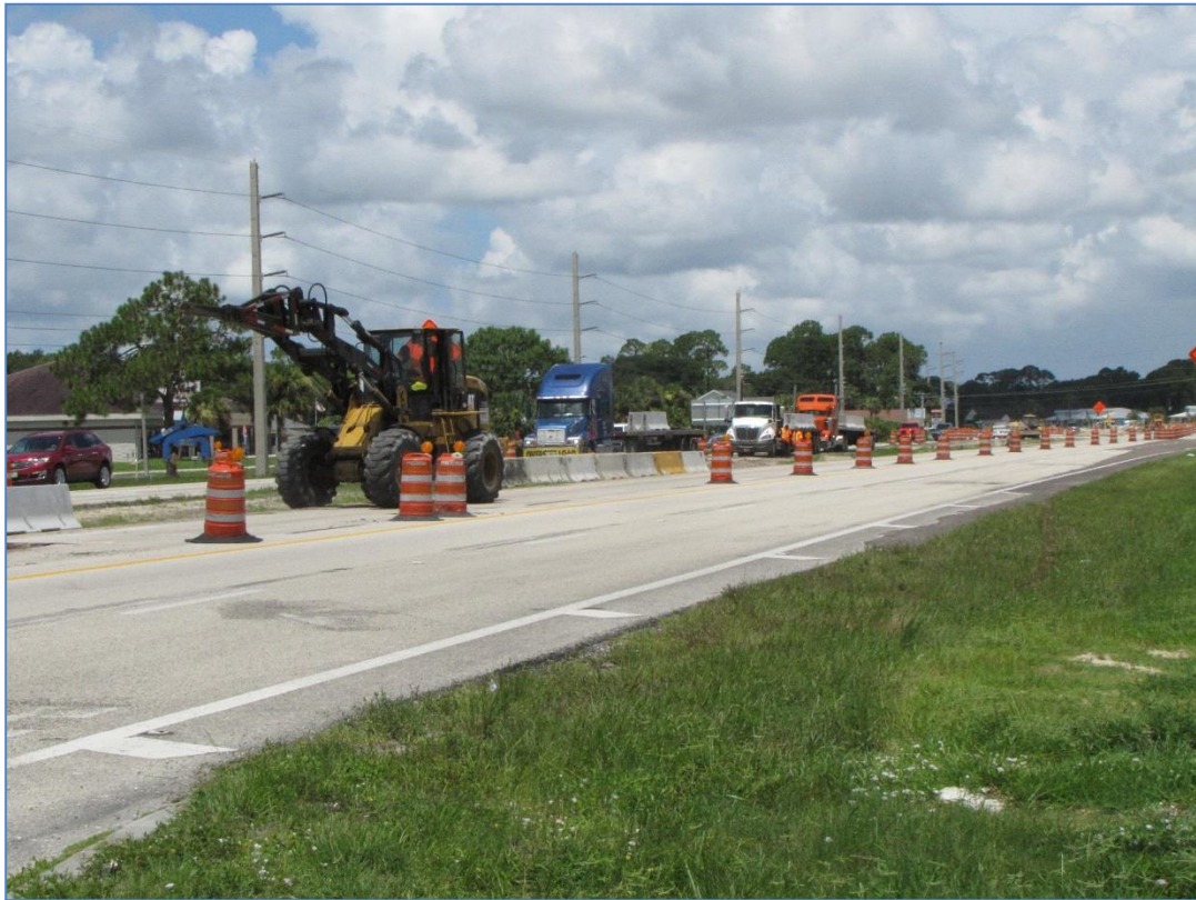
U.S. 41 Six-laning project in District One
