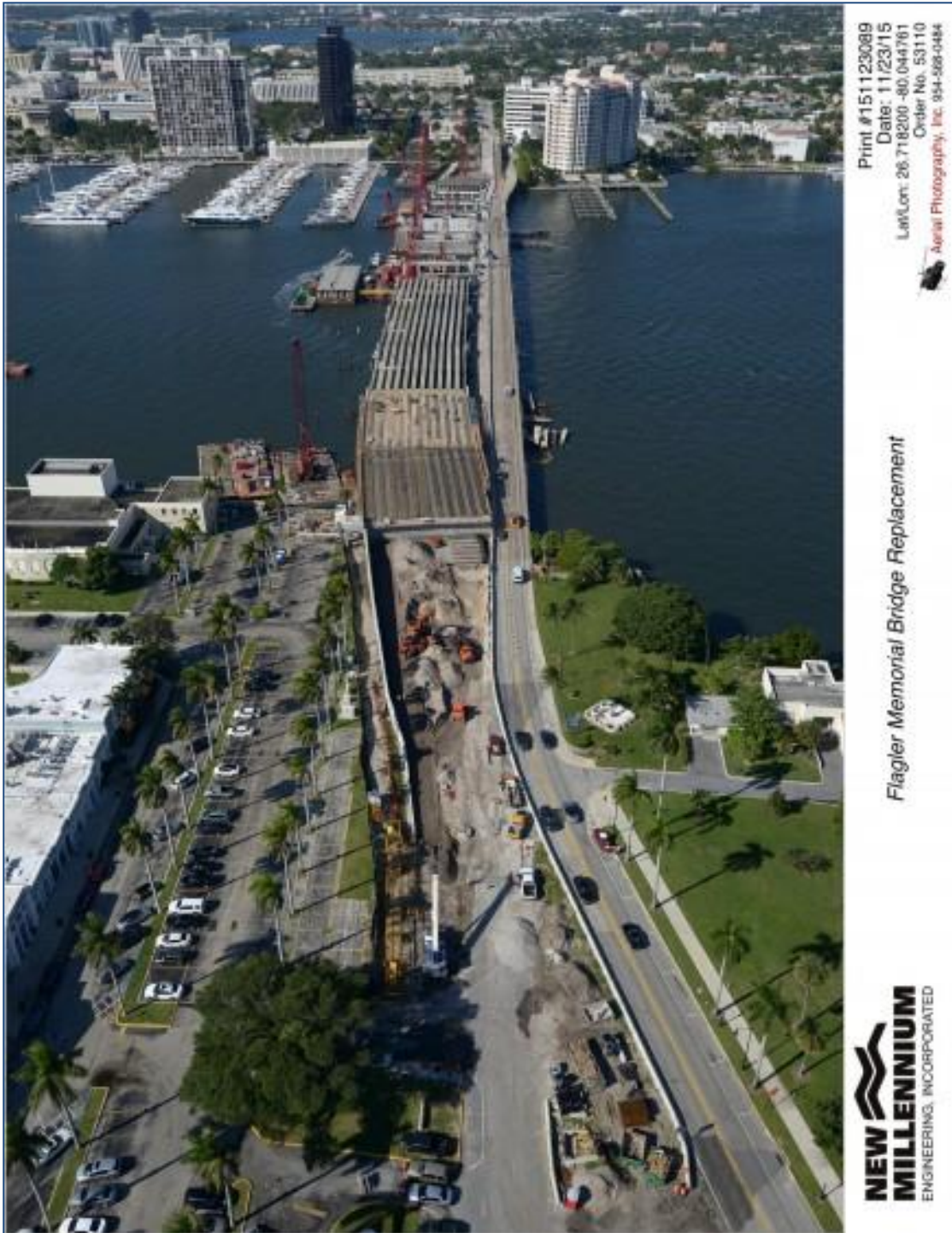
Flagler Memorial Bridge Replacement in Palm Beach County.
